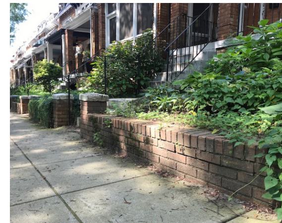
The front yards of most Kingman Park rowhouses are retained by low brick walls.
