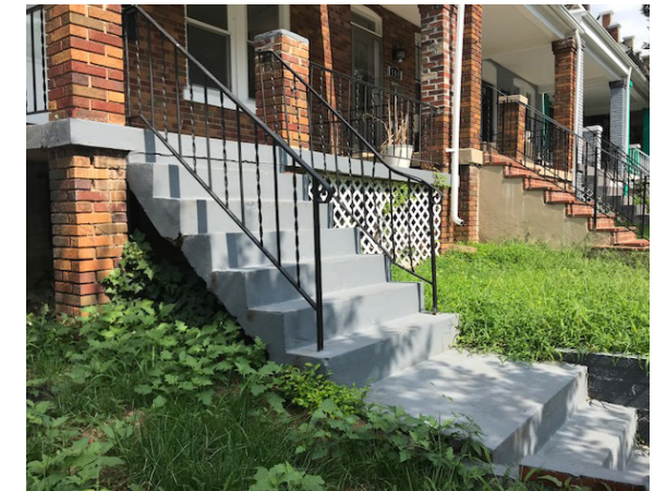
The front Lead walks and stairs are smooth concrete.
