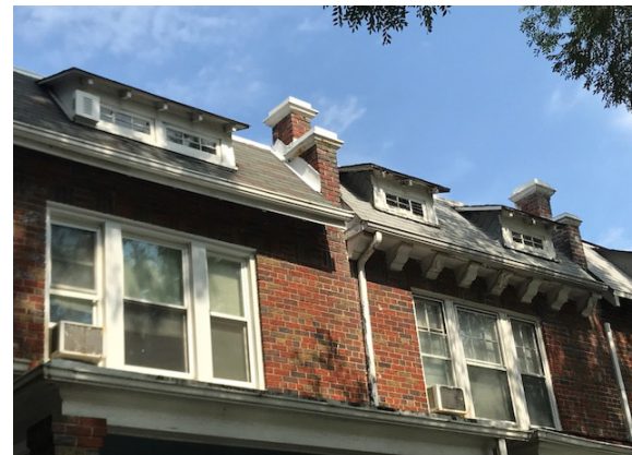
Rowhouse roofs with overhanging eaves, cornices, dormer windows and parapet walls on the sides.
