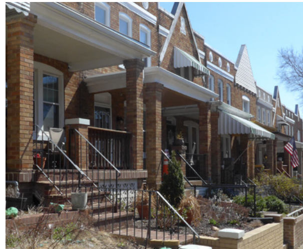
Front porches with brick piers.
