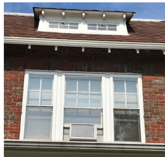
Original second floor and dormer windows.
