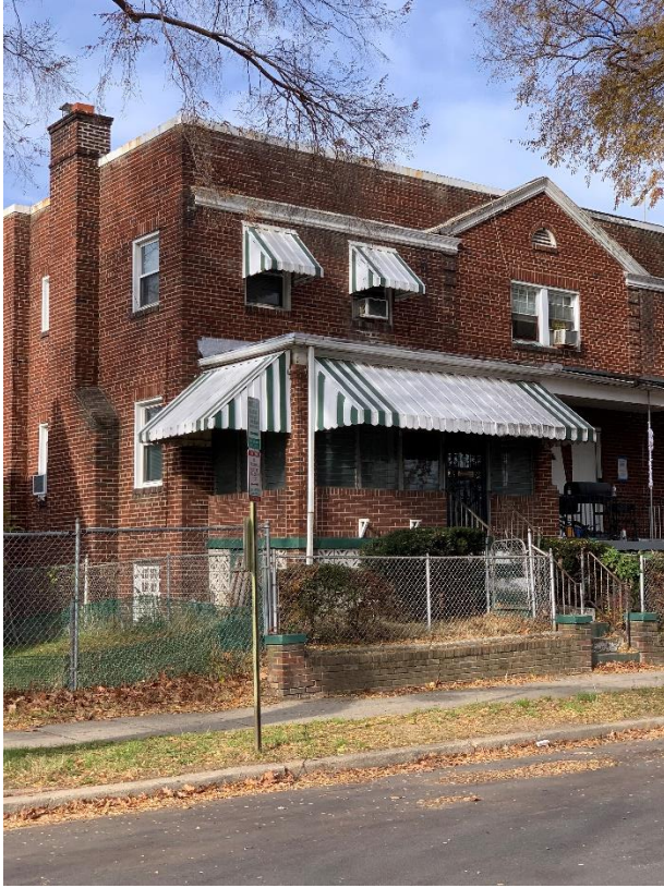
View looking northwest from center of 23 rd Place NE south of 406 23 rd Place NE (with center gable). Mock-up not visible.
