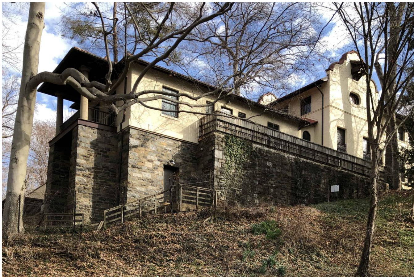
Photo 9: House of Mercy, South Wing, Rear Extension (J. DeFerrari).
