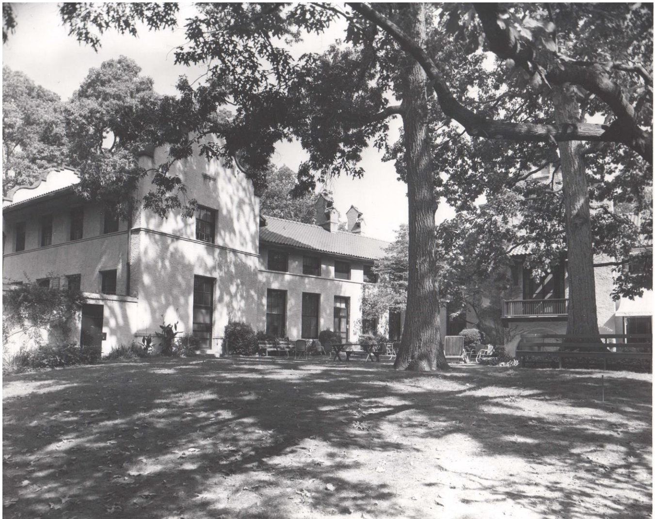
Photo 3: Undated historical view of the courtyard of the House of Mercy (Rosemount Center archives).
