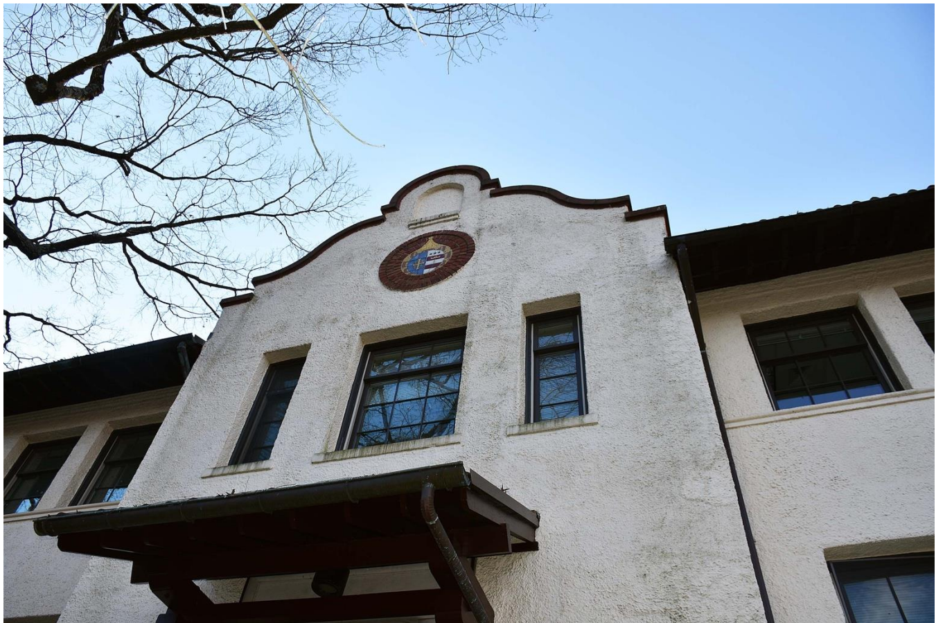
Photo 6: House of Mercy, Front Façade Parapet detail (D.P. Sefton).
