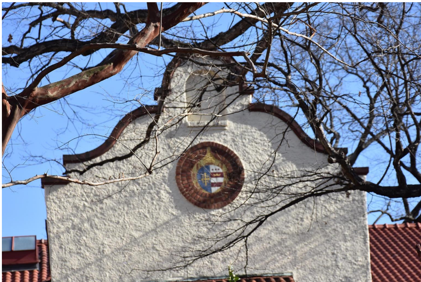
Photo 14: House of Mercy, Main Block Rear Façade, Parapet detail (D.P. Sefton).
