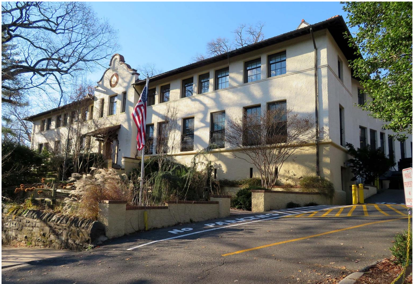
Photo 5: House of Mercy, Front (East) Façade from Rosemount Avenue NW (J. DeFerrari).
