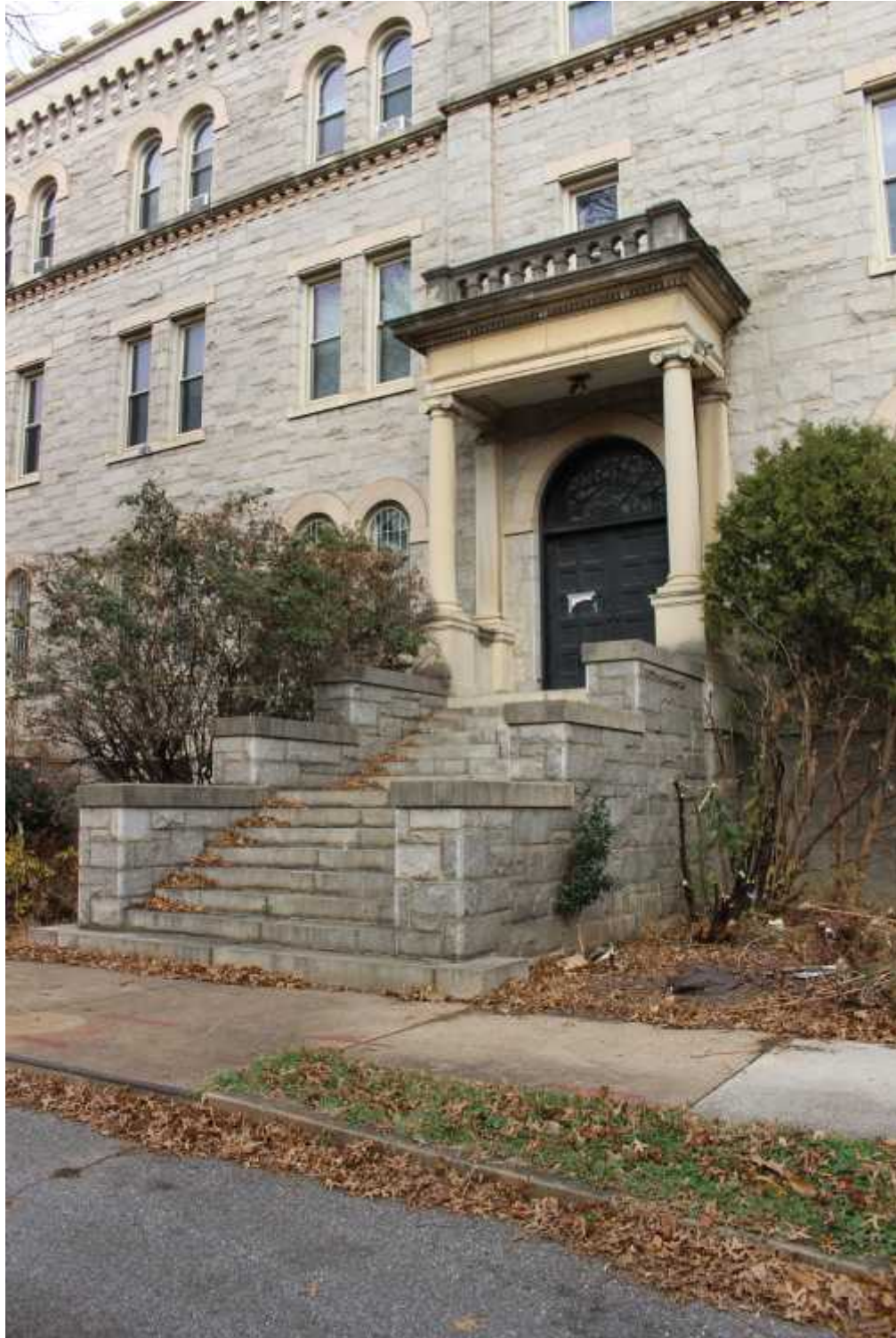
9 of 20 South entrance, facing northwest
