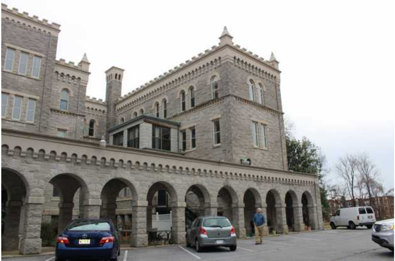
6 of 20 West (rear) elevation, facing southeast
