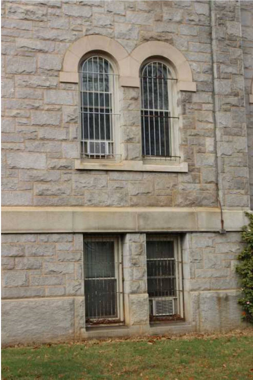
10 of 20 Typical basement and first-story windows on front elevation, facing west
