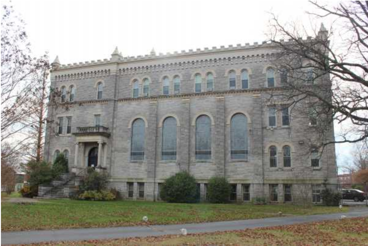
2 of 20 North (side) elevation, facing south
