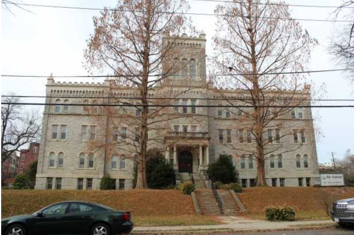
1 of 20 Front (east) elevation, facing west
