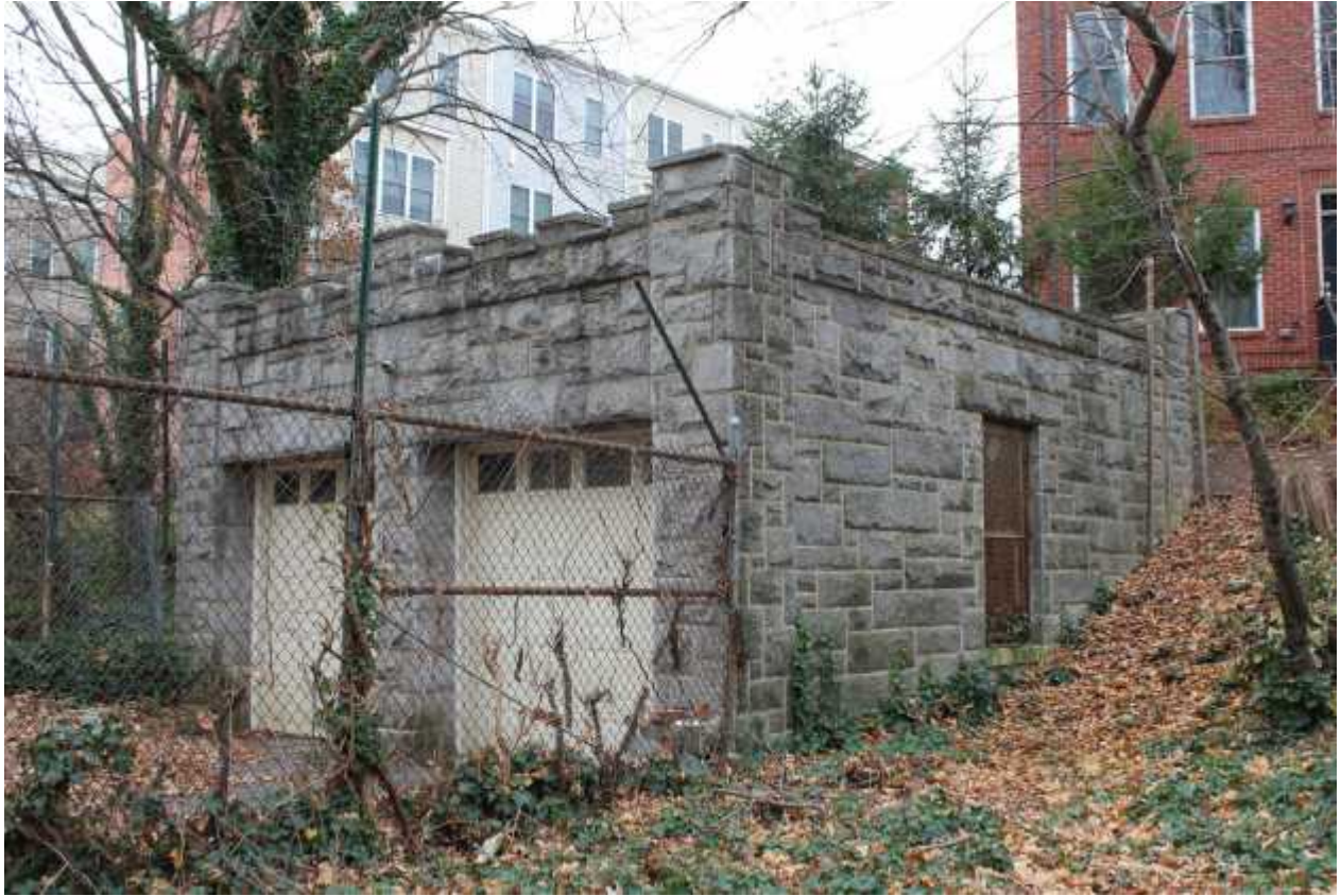
15 of 20 Garage, facing southwest
