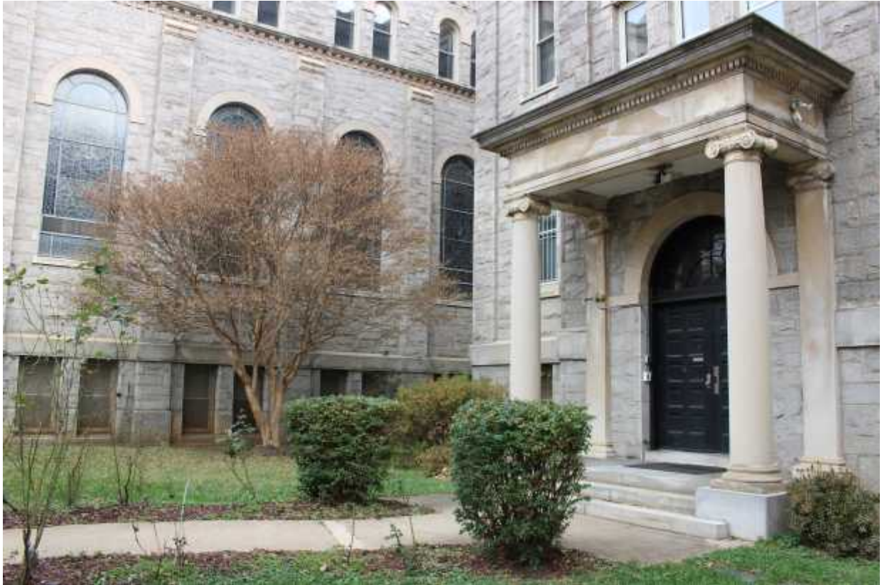
13 of 20 Rear courtyard with entrance, facing northeast
