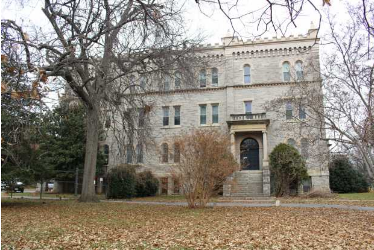
3 of 20 South (side) elevation, facing north
