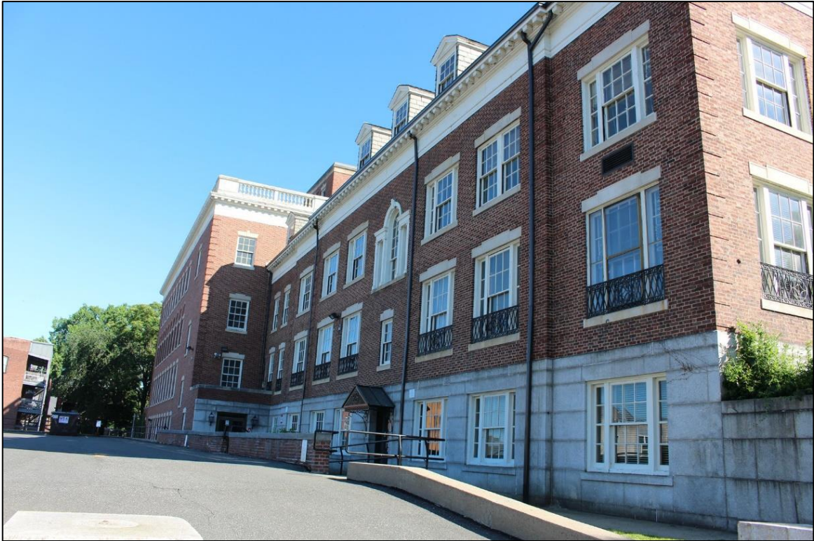
2. South and East Elevation Elevations of 1924 Bank Building and 1935 Addition, looking north.
