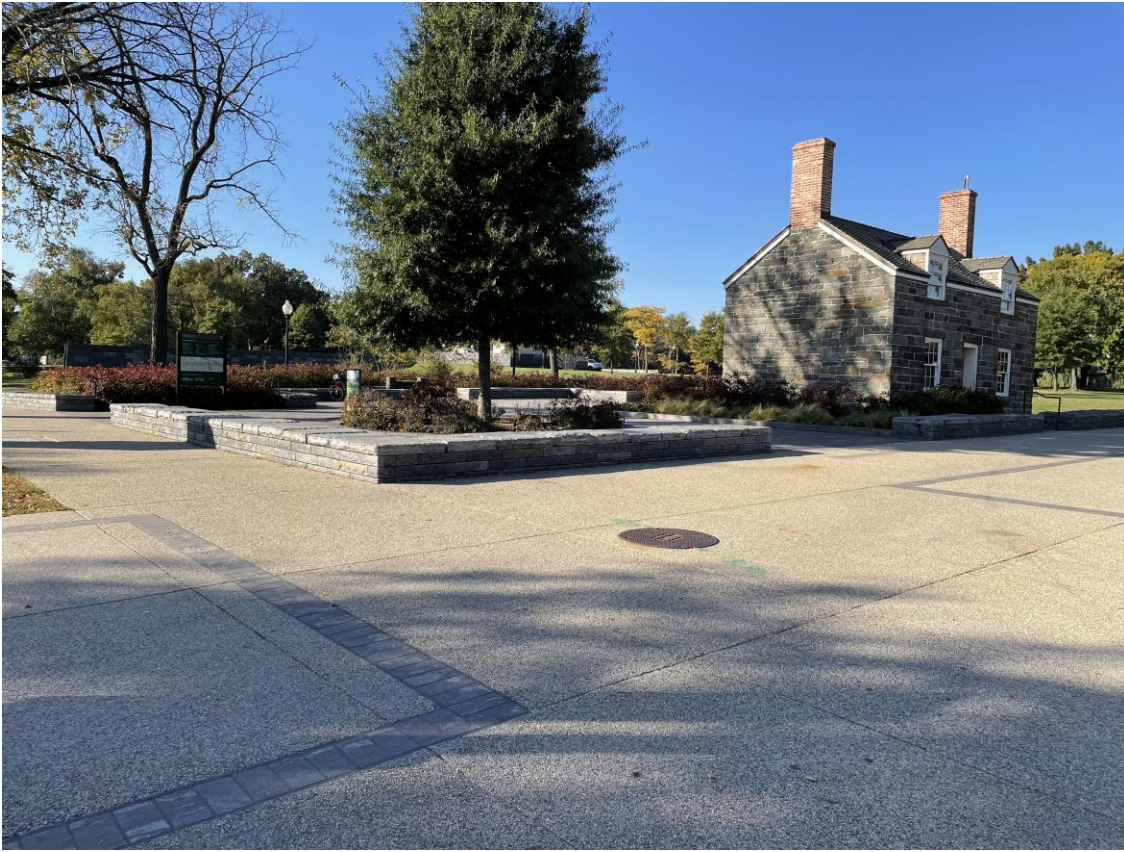
View looking SW from 17 th Street and Constitution Avenue showing the Washington City Canal Lockkeeper's House on its new site within a landscaped plaza area. The original 1837-1915 location of the building, demarcated by dark-colored stone pavers, is visible at the left of photograph and the 1915-2017 location of the building similarly demarcated is visible at right of the photograph.
