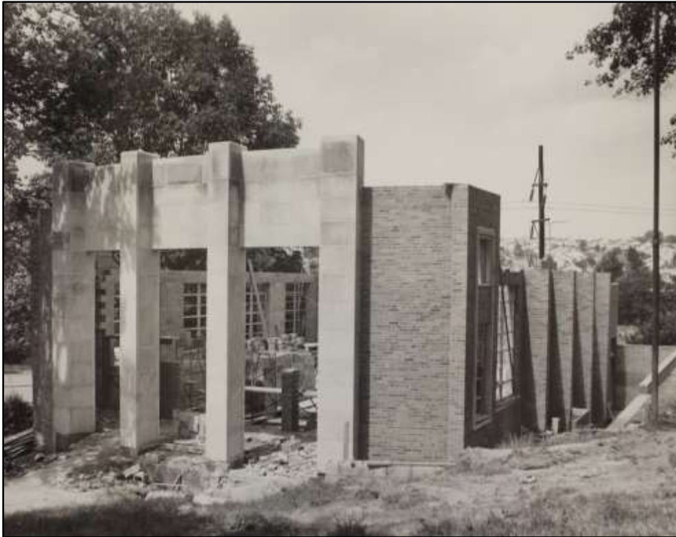
c.1961 photograph of the National Memorial Chapel under construction ( Library of Congress, Prints and Photographs Division, Nannie Helen Burroughs Collection, Lot 12571, Location G, Box 2 of 2 ).
