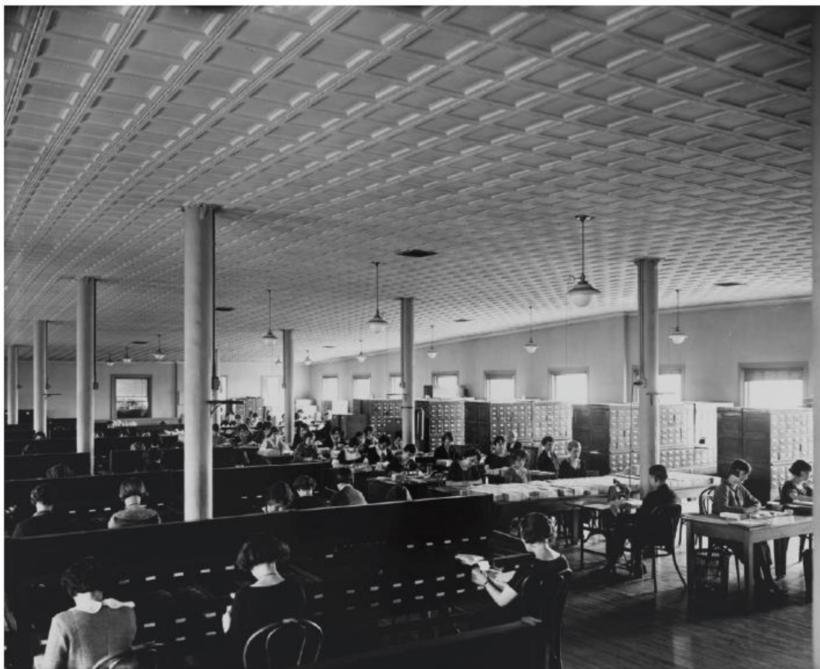
Figure 2.3 Upper level of the Chas. Lesser's Randolph Place Building showing Arthur Heaton's renovations and NGS staff at work. Photo Credit- Edwin I. Wisnerd / National Geographic Creative
