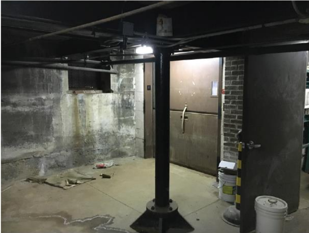
Figure 3.29 Steel Column at Basement of Schlitz Building
