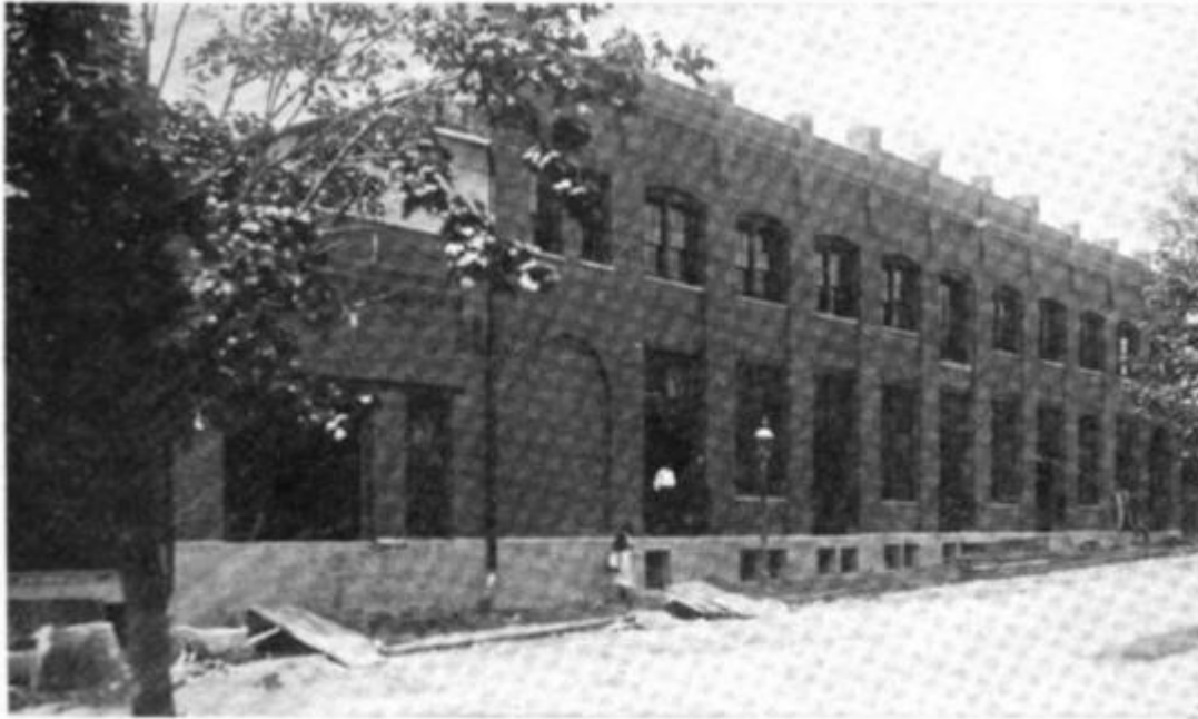
Bottling Works, Schlitz Brewing Co. Washington, D. C. Chas. L. Lesser, Milwaukee, Wis., Architect. J. M. Dunn, Washington, D. C., Contractor. Universal Portland Cement Used
