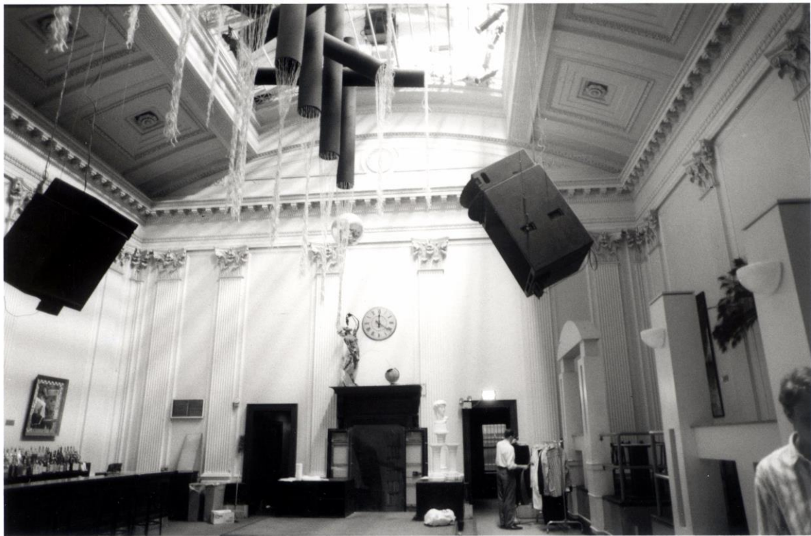
Figure 1. Banking hall, north wall. Earliest known photo of interior, 1989
