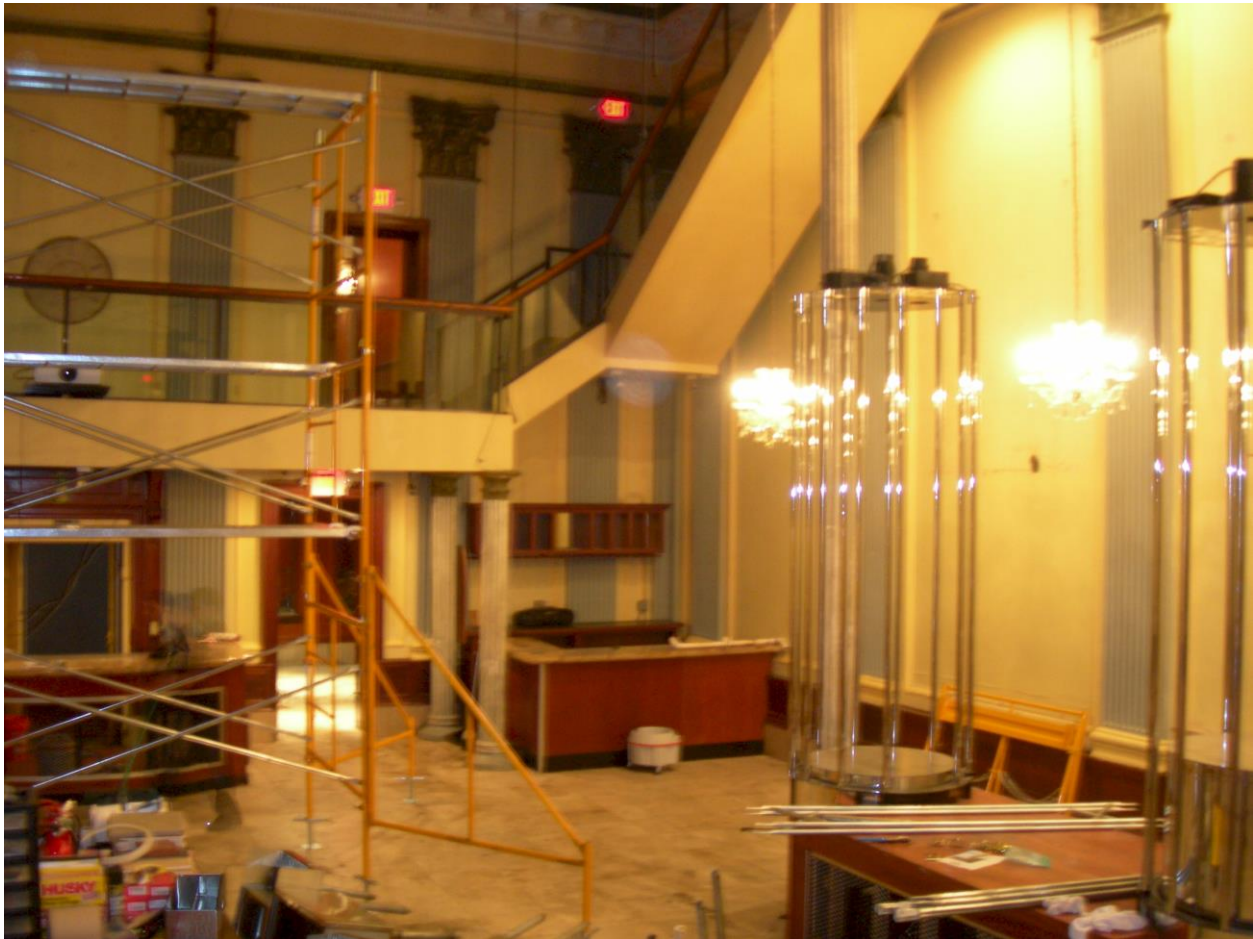
Figure 2. Banking hall, northeast corner, mezzanine and catwalks prior to removal in 2010.
