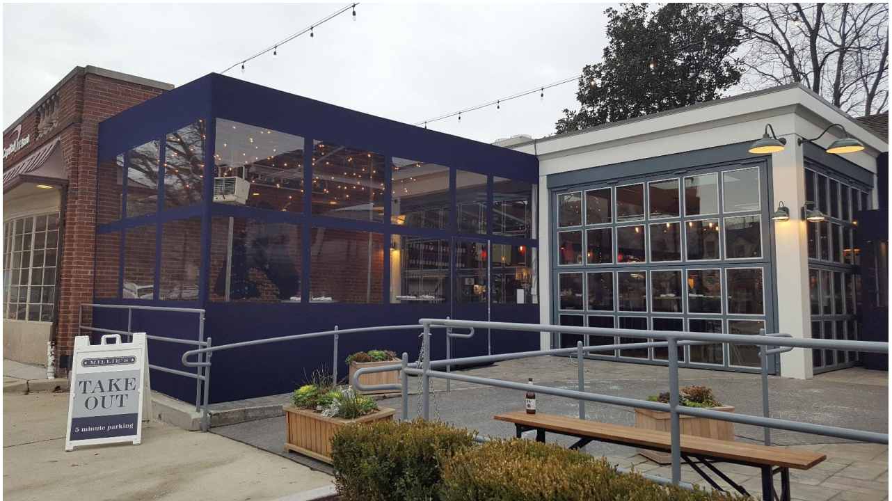
Temporary seasonal enclosure at 4866 Massachusetts Avenue NW
