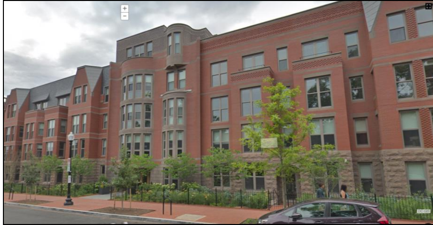
New construction, 8 th Street SE, Capitol Hill Historic District
