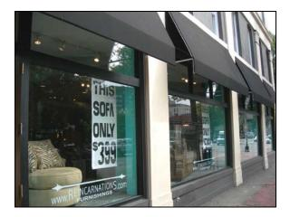
Awnings and canopies should be made of treated, weather-durable fabric such as canvas or woven acrylic. Vinyl, metal, and plastic are not appropriate awning or canopy materials.
