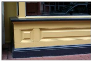
Typically made of wood or masonry, window bases are sometimes surfaced with metal panels, ceramic tiles, marble, brick, or other materials.
