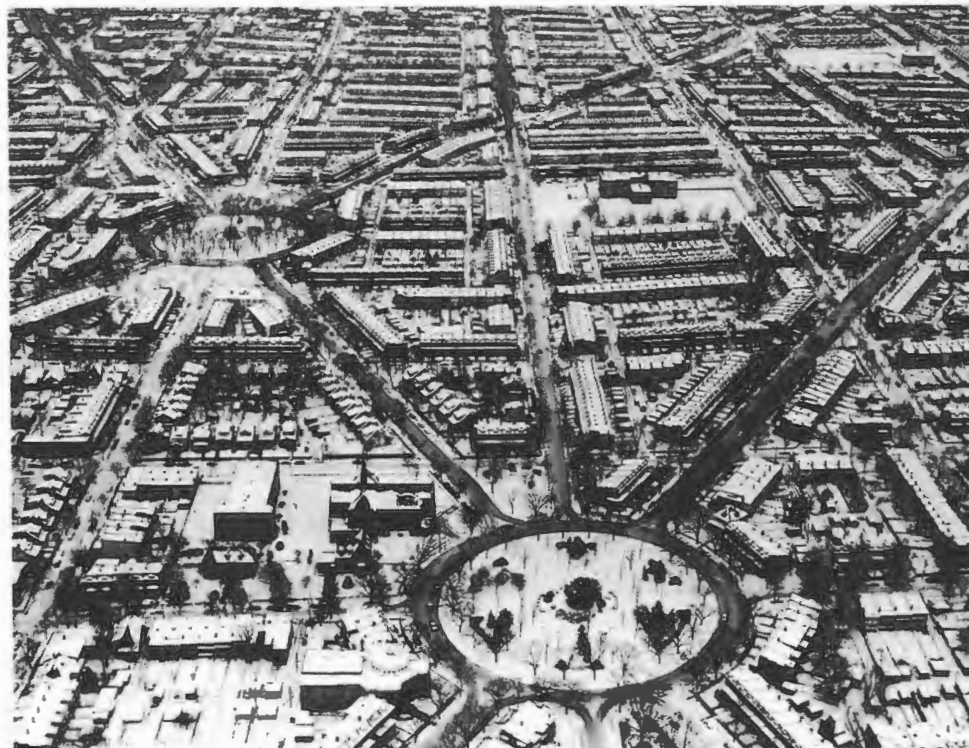
1954 Aerial Photograph over Grant and Sherman Circles
