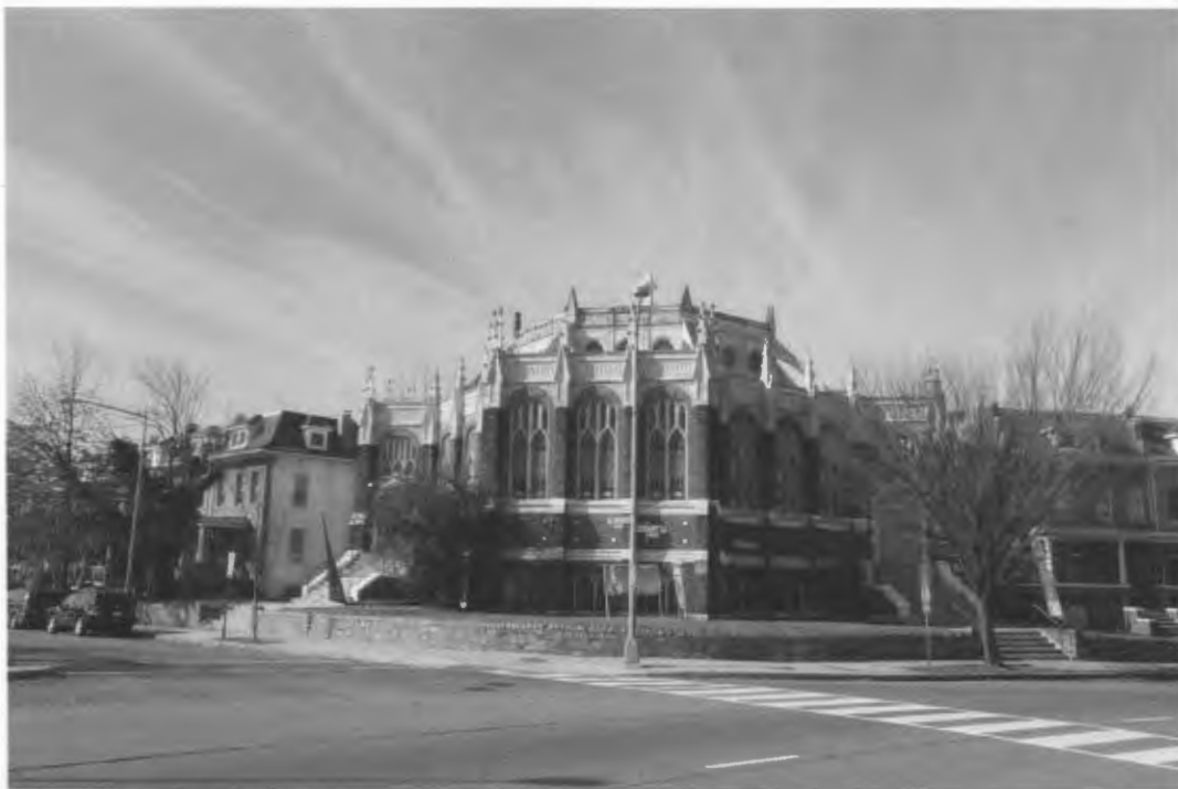
Photo 19 of 26: DC_Grant Circle Historic District_019.tif Petworth United Methodist Church, 33 Grant Circle, facing west
