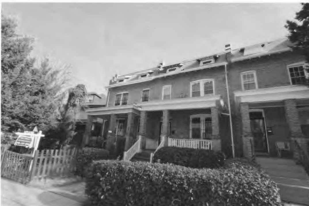
Photo 6 of 26: DC_Grant Circle Historic District_006.tif 13-15 Grant Circle, facing east
