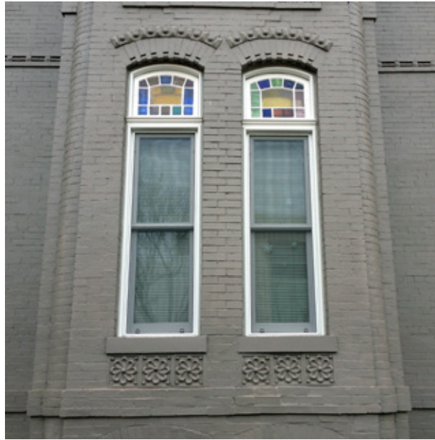
Appropriately replaced windows and restored original transoms at Klipstine Row, 526 22nd Street NW
