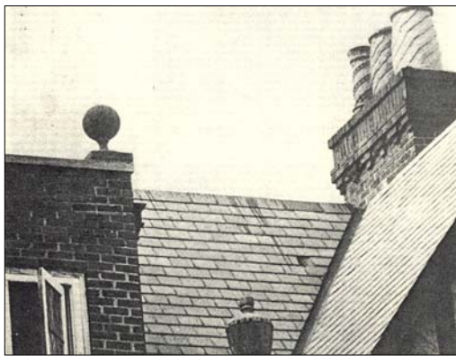
Any installation on a roof should not result in the loss or alteration to distinctive architectural features such as shingles, chimney pots, or other decorative details.
