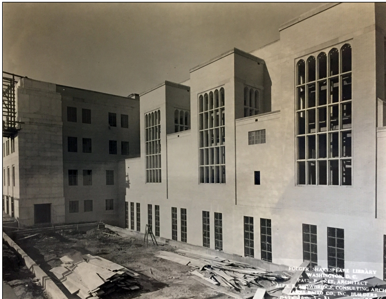
Figure 24. South (rear) elevation of the Folger Library under construction, January 1931 (Folger Archives)
