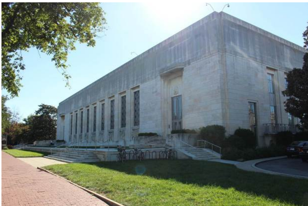
Photo #0001: DC_Washington_Folger Shakespeare Library_0001.tif North elevation, looking east
