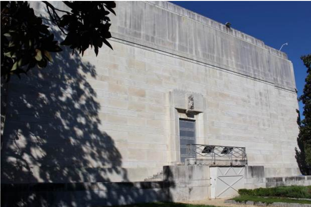
Photo #0005: DC_Washington_Folger Shakespeare Library_0005.tif East elevation, looking northwest.
