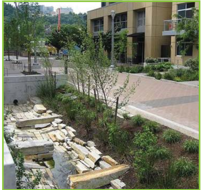
Figure 33: Vegetated Filter Strip
