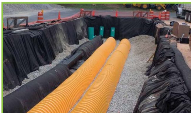
Figure 27: Underground Storage Facility
