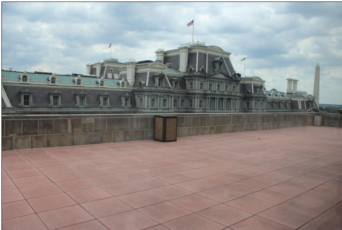
6th Floor Terrace, Looking Southeast
