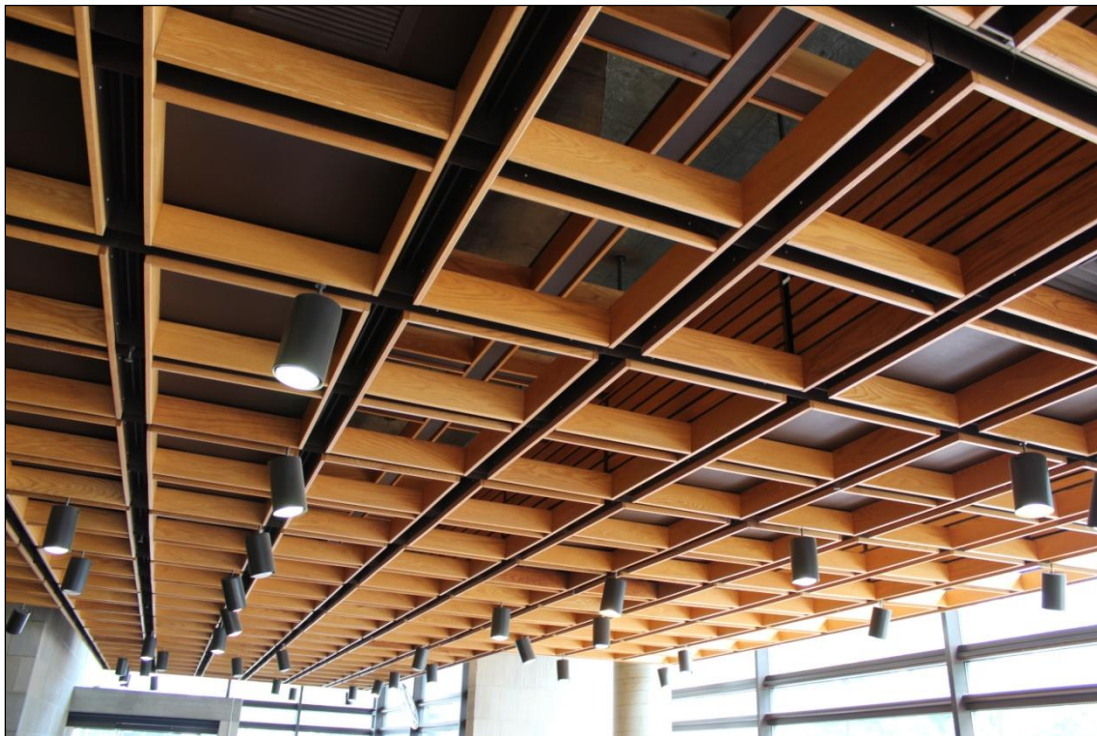
FHLBB Building Wood Drop Ceiling in Lobby, Looking NE
