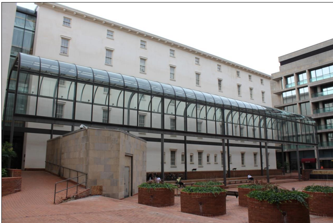
The Galleria, Looking SW
