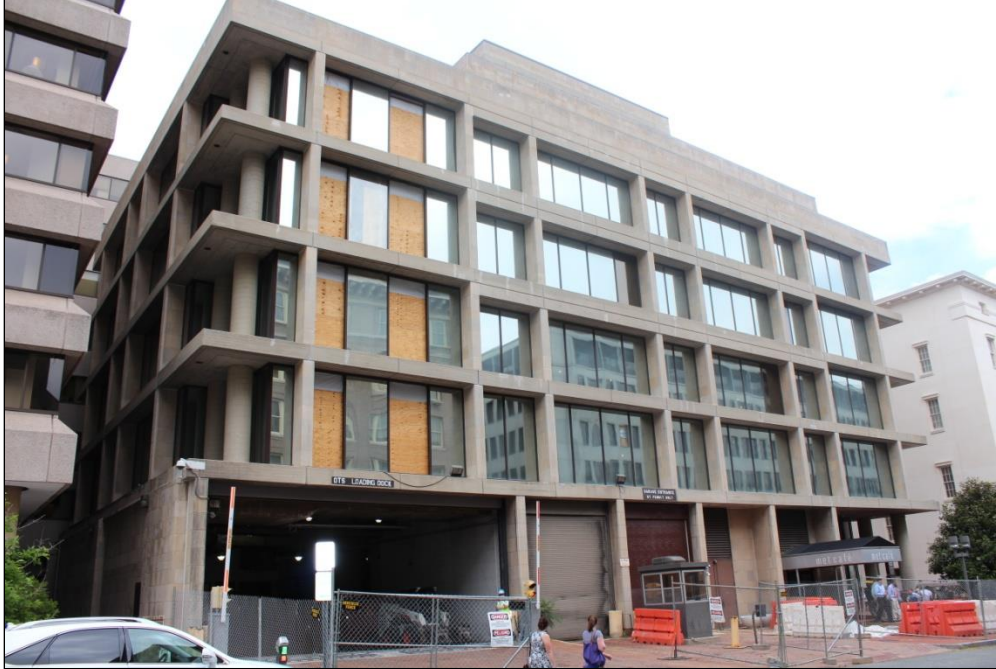
FHLBB Building, South Elevation of South Wing, Looking NE
