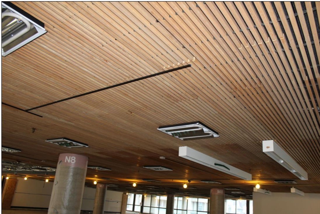
Detail of Wood Slotted Ceiling on Fifth Floor, Looking SW
