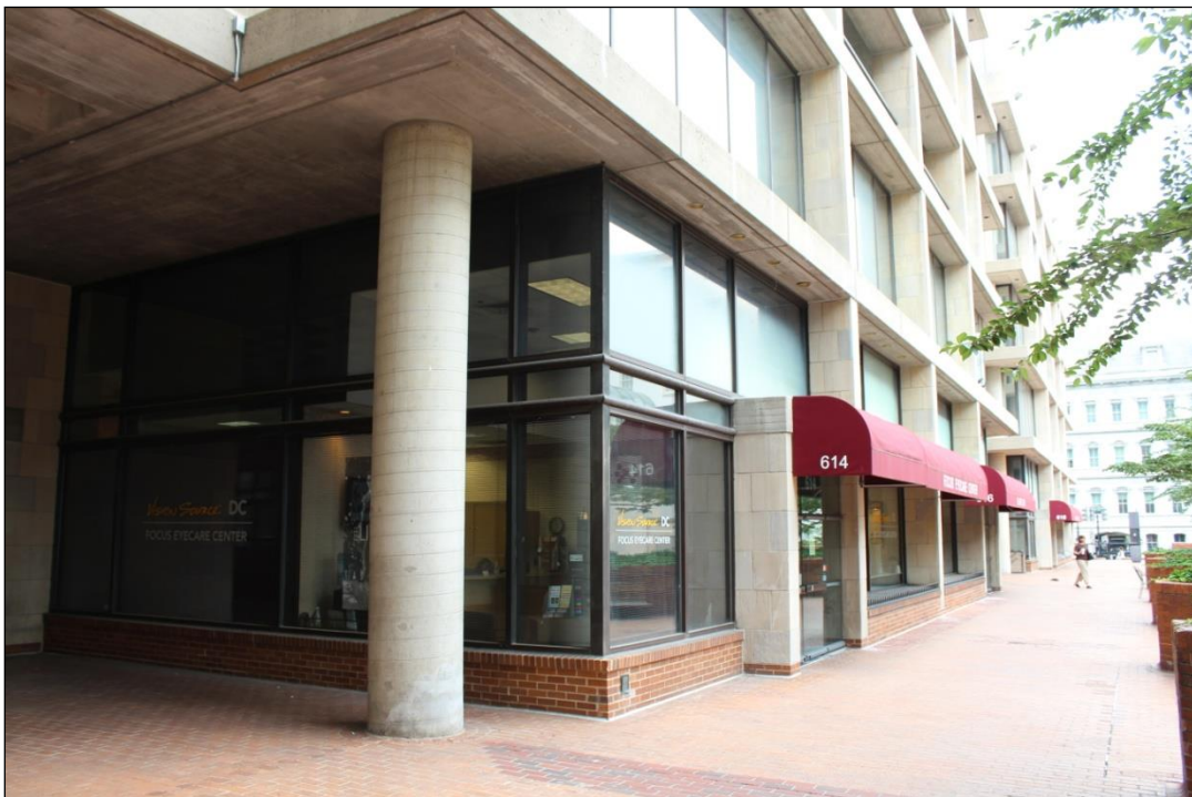
FHLBB Building, Detail of Storefronts on South Elevation of East Wing, Looking NE
