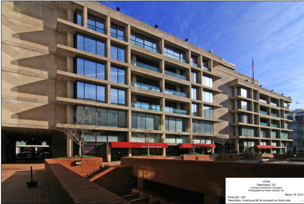
FHLBB Building, South Elevation of East Wing, Looking NE
