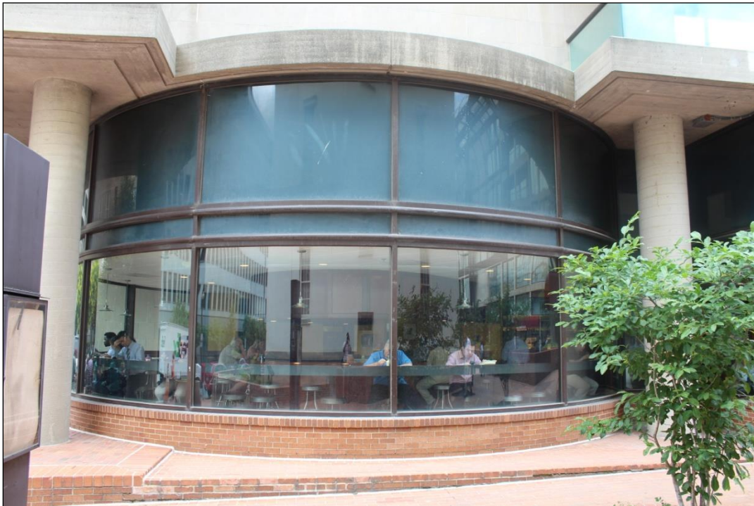
FHLBB Building, Circular Bay on East Elevation of South Wing, Looking West
