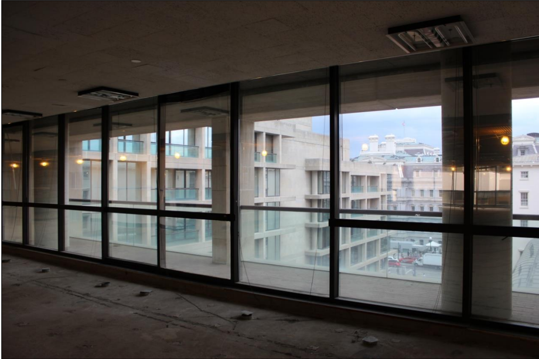
Balconies on Fifth Floor, Looking NE
