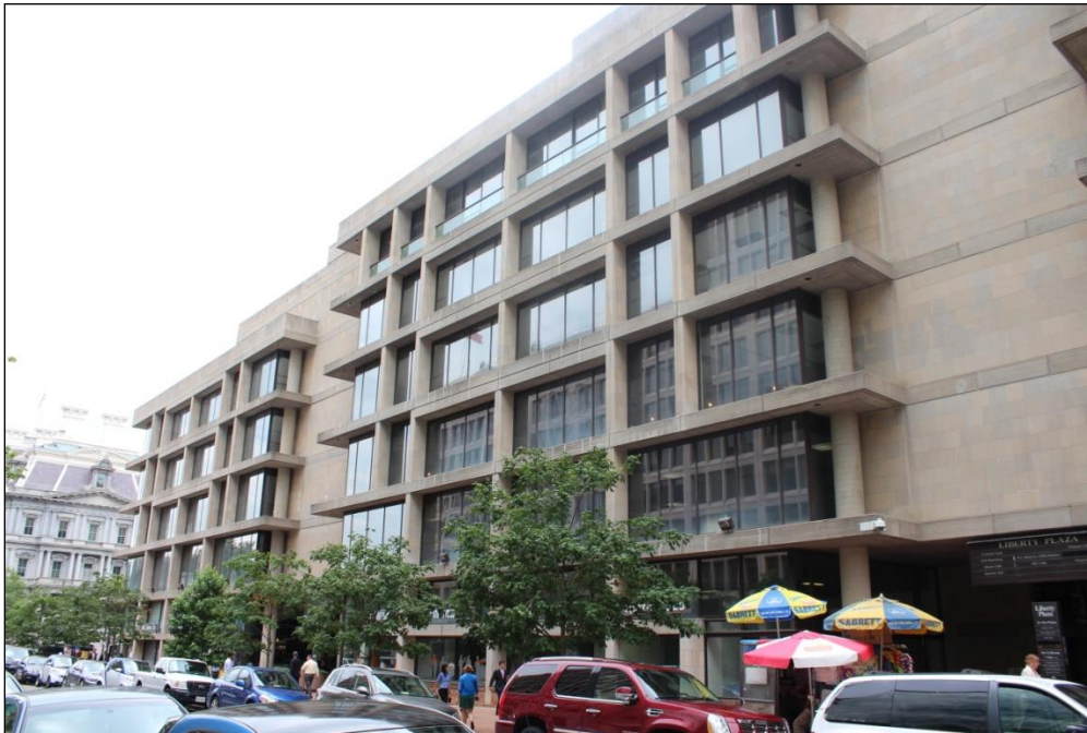
FHLBB Building, North Elevation of East Wing, Looking SE
