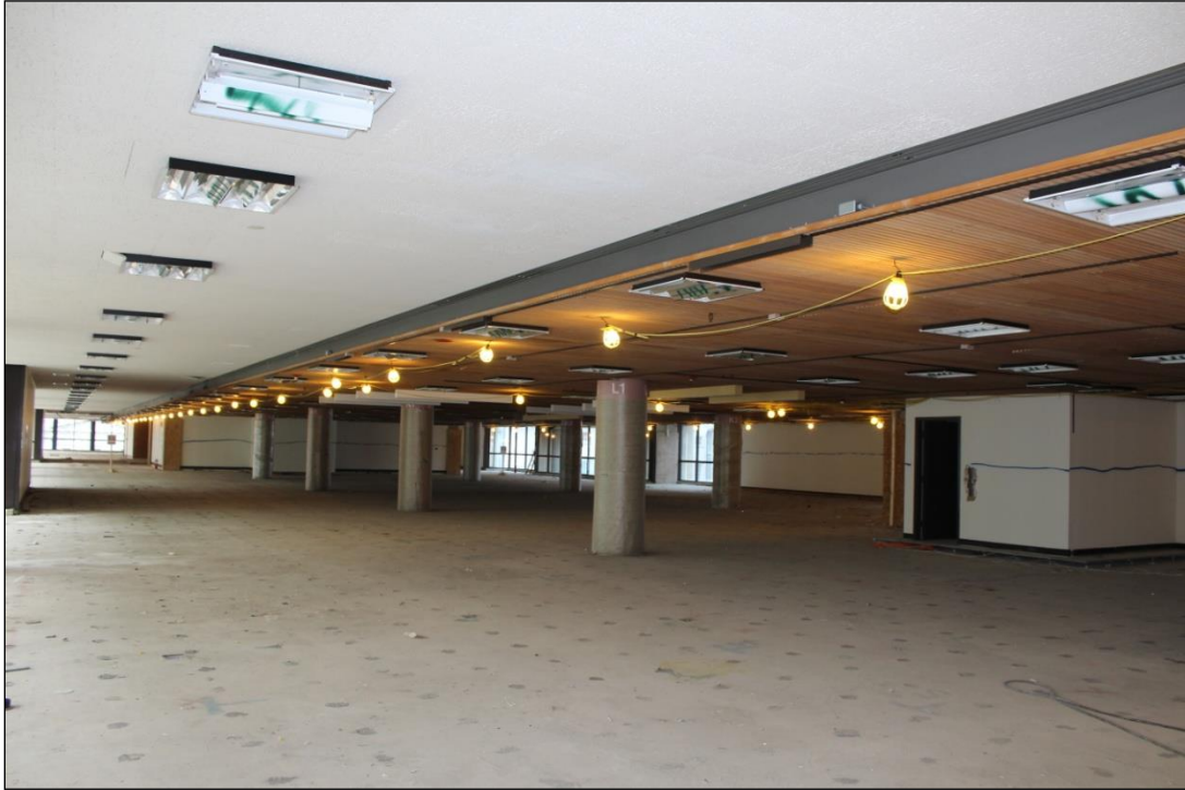
Fifth Floor, Looking Southeast
