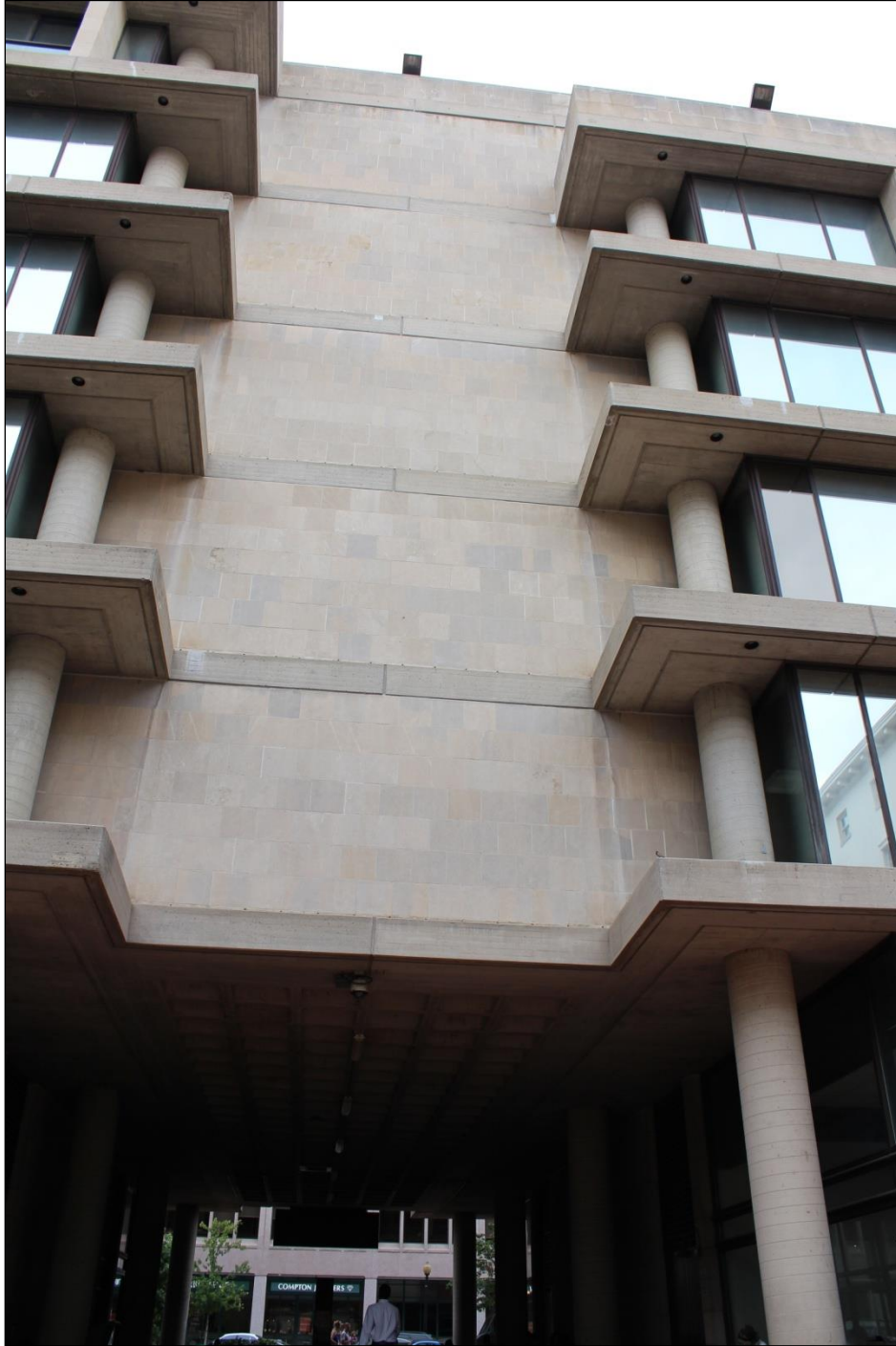
FHLBB Building, Detail Limestone Exterior, Looking North from F Street
