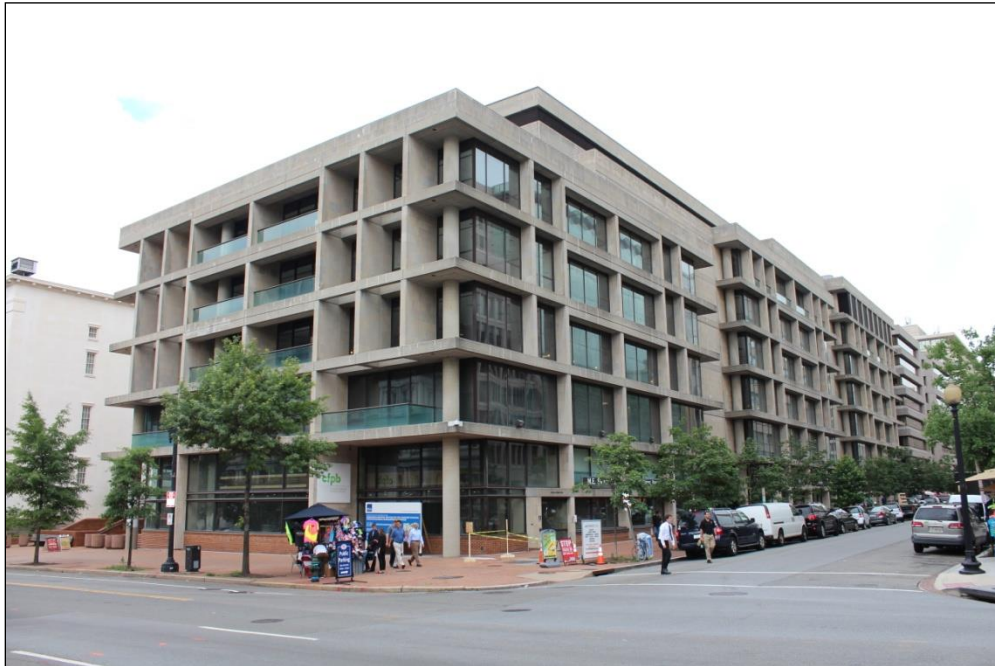
FHLBB Building, North and East Elevations of East Wing, Looking SW
