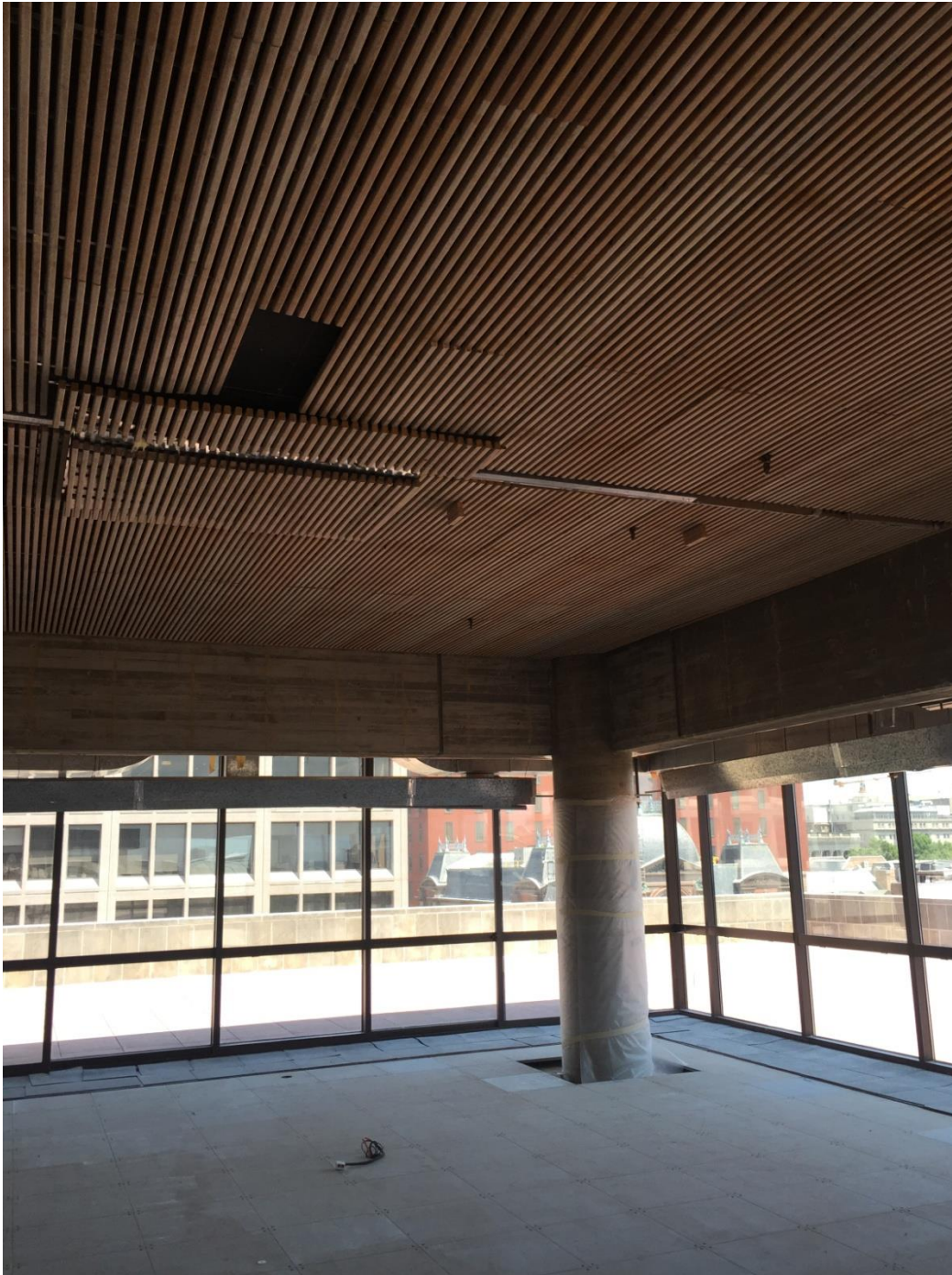
Sixth Floor East Side of Building, Looking SE
