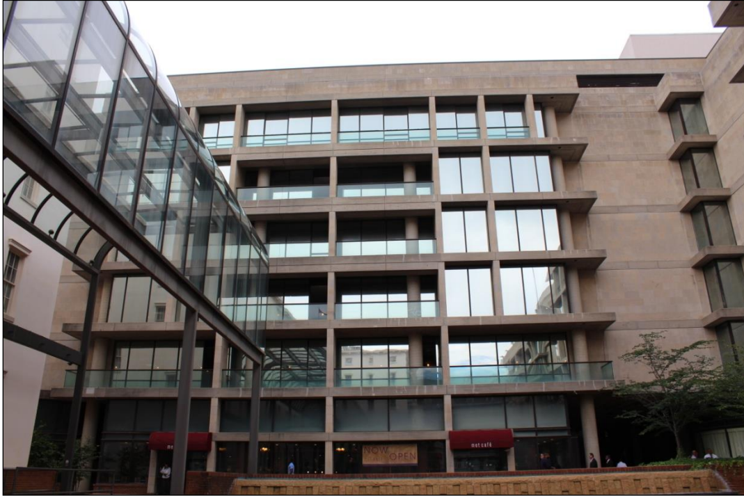
FHLBB Building, East Elevation of South Wing, Looking West
