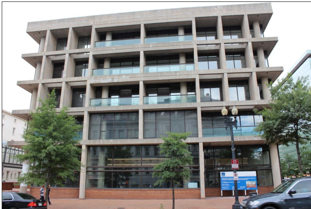
FHLBB Building, East Elevation of East Wing, Looking West
