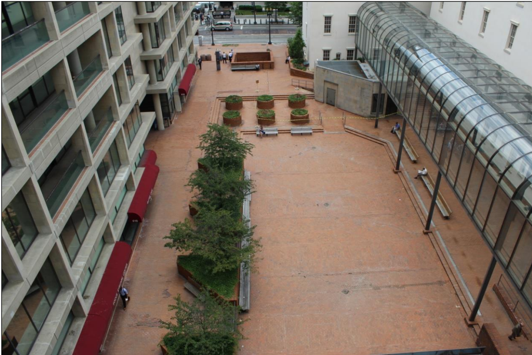
Liberty Plaza, View from 6th Story of FHLBB Building, Looking East
