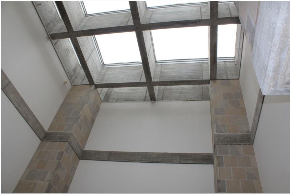
6th Floor Atrium in South Wing
