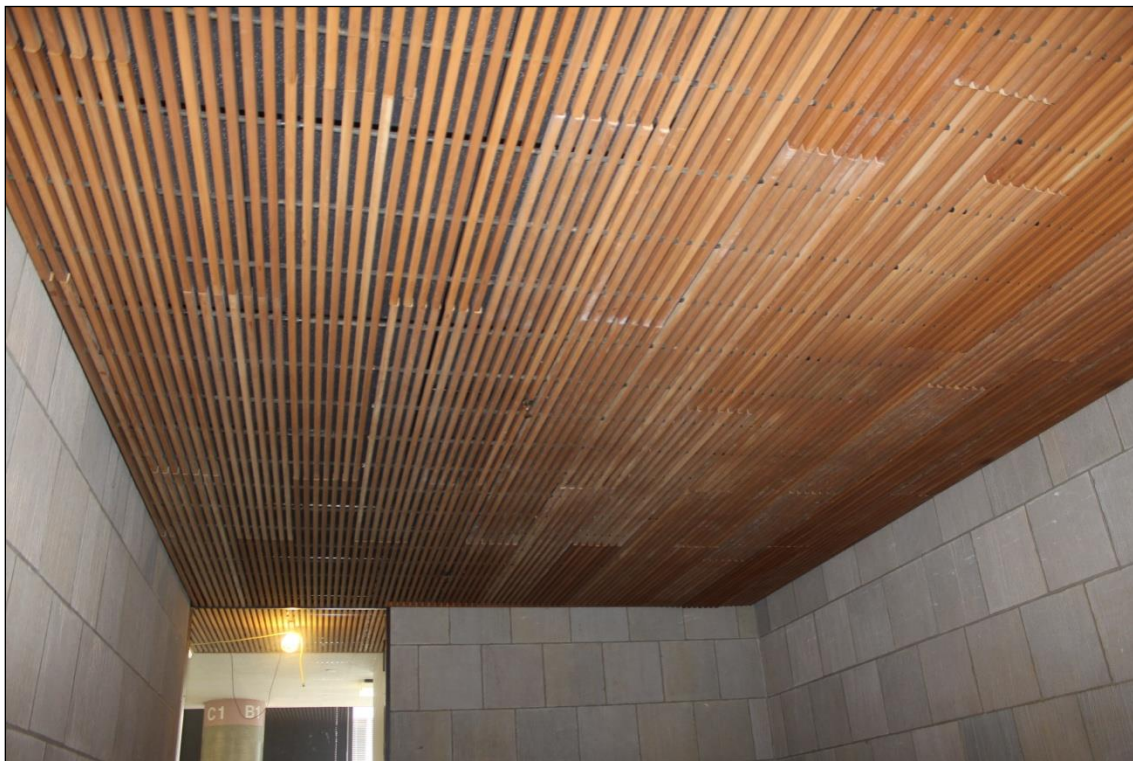
FHLBB Building, Slot Wood Ceiling in High-Bay Portion of East Lobby, Looking North
