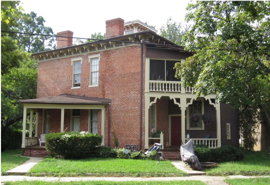
The Jost-Kuhn Farmhouse at 1354 Madison Street was once the center of a 24-acre farm. The house sits slightly askew to the street and is readily recognizable as an historic farmhouse among the mid-20 th century neighboring houses.
