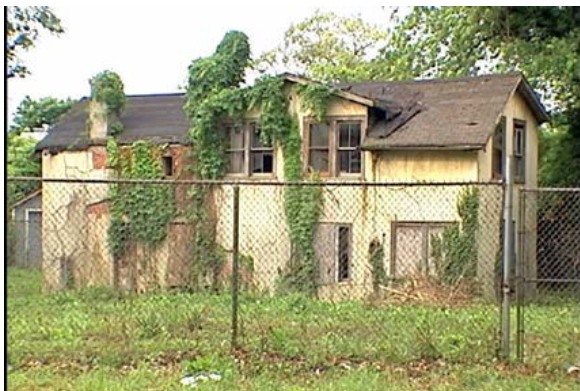
This barn, historically part of the 24-acre Jost-Kuhn Farm, stood until 2004 before being demolished. Only two barns survive in the city: the Peirce Barn and the Barn at Saint Elizabeths.
