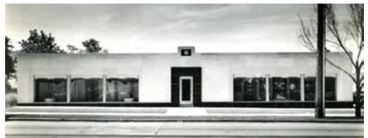
PEPCO SUBSTATION NO. 38
