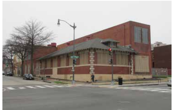
PEPCO SUBSTATION NO. 13
