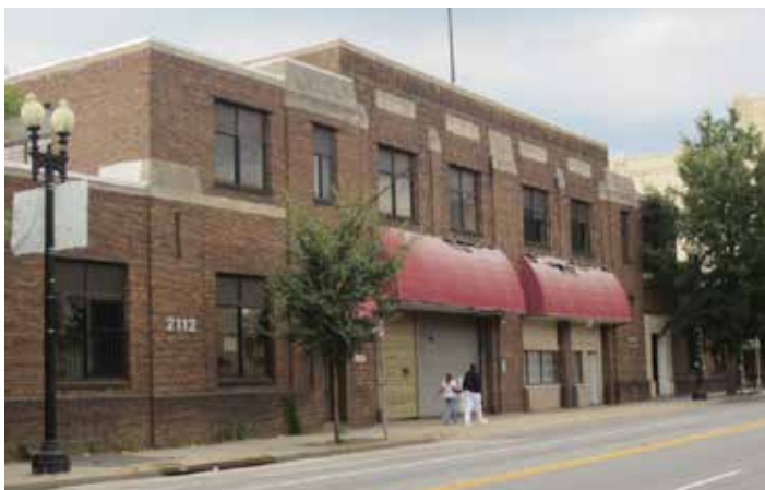
WASHINGTON RAILWAY AND ELECTRIC COMPANY GARAGE
