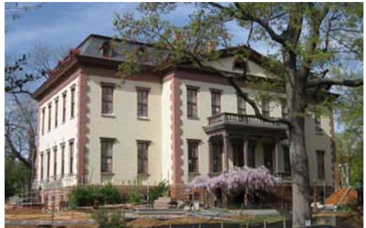
OLD NAVAL HOSPITAL, BEFORE AND AFTER
