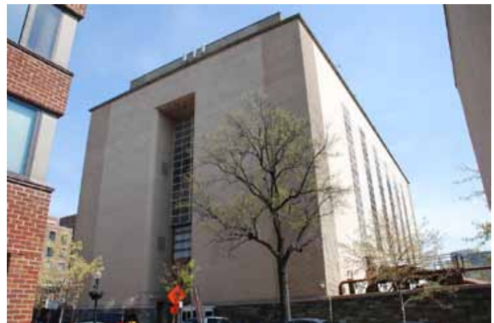
WEST HEATING PLANT
