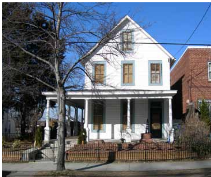
1420 W STREET, SE, AFTER
