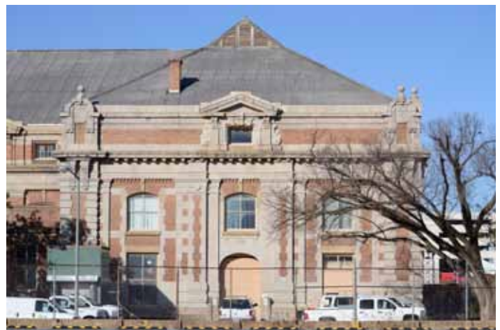
MAIN SEWERAGE PUMPING STATION
