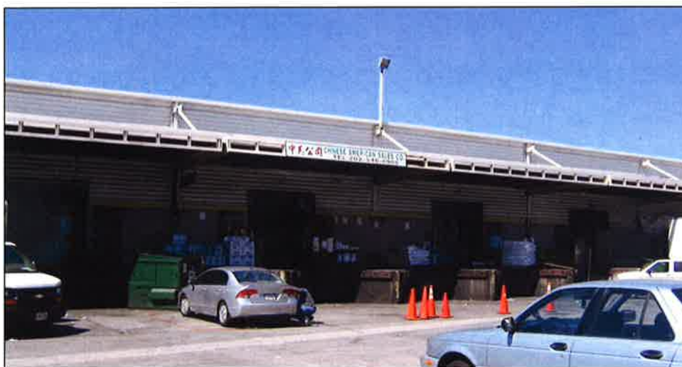
Figure 15: Market Building Constructed in the 1980s (photo from 2007)
