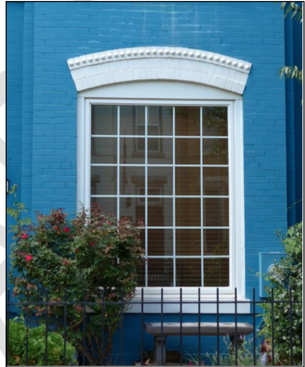
This window installation resulted in the loss of original decorative framing elements.
