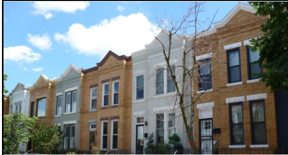
Decorative cornices and parapets characterize the roofline of Emerald Street houses.
