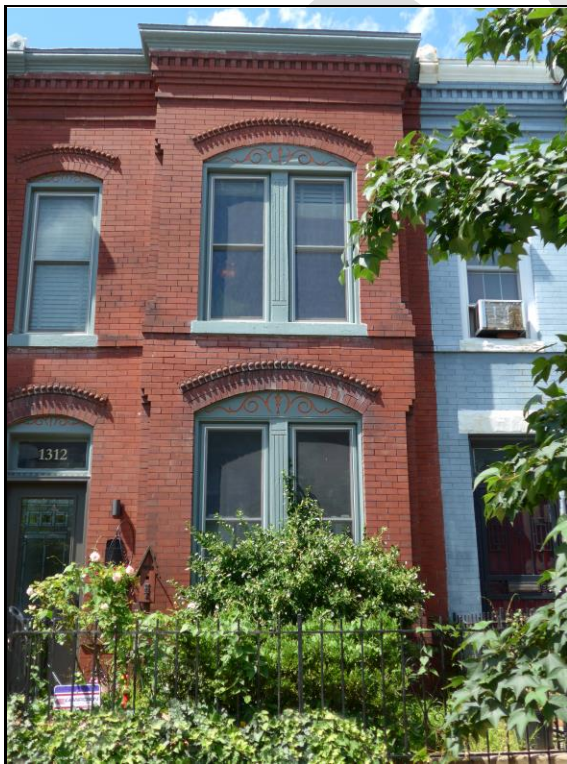
The replacement windows on this house replicate the originals. The installation maintains the decorative fluted muntin and lunette panel with ornamental scroll-sawn detailing above.
