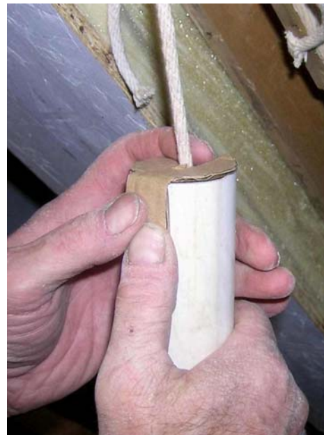
Cardboard in place over PVC tube
