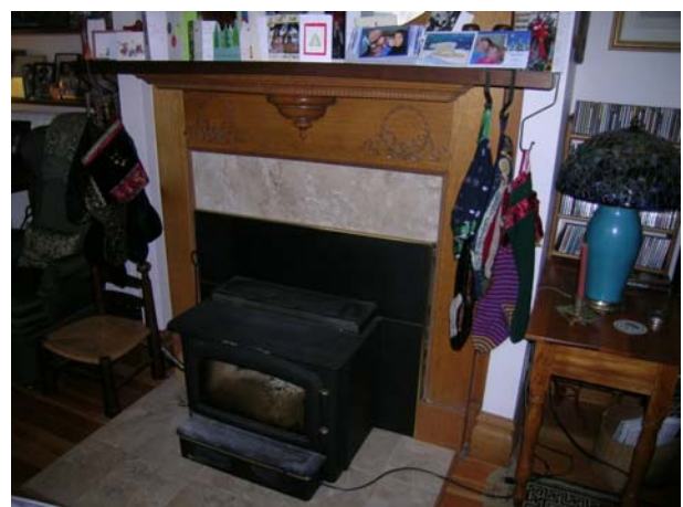
Wood stove vents into existing chimney
