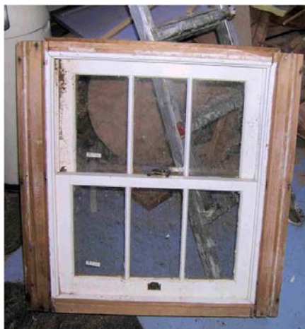
Old window with closed counter weight pockets
