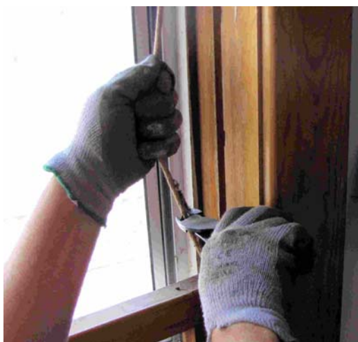
Figure 3-5. Repairing rope system
