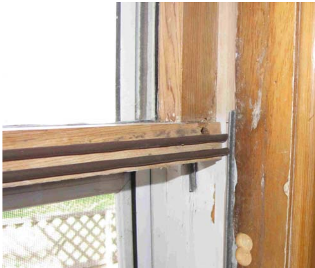
Figure 3-7. Retrofit of parting rail with weather strip
