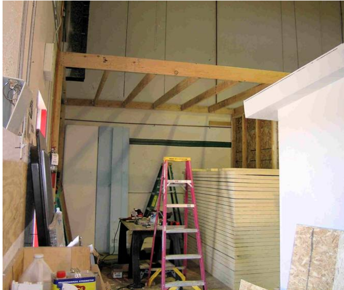
The chamber was framed into the corner of a warehouse. The existing walls were first covered in two inches of polyisocyanurate (R-13).
