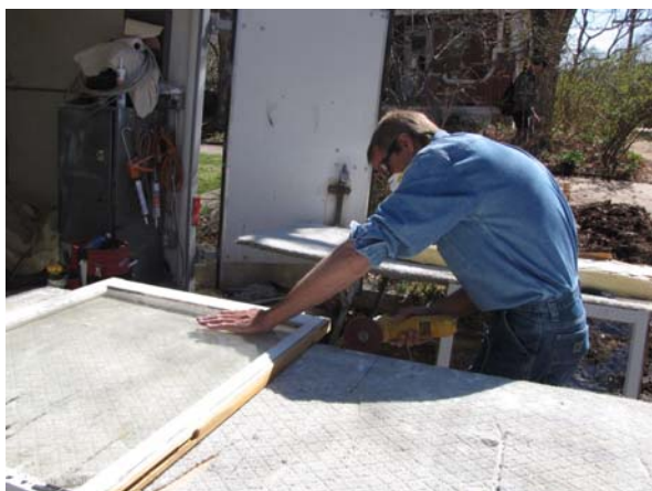
Figure 3-4. Sanding the window
