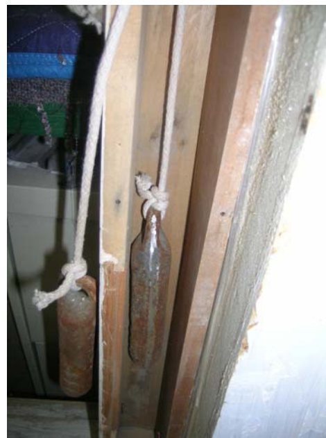
Open pocket with counter weight
