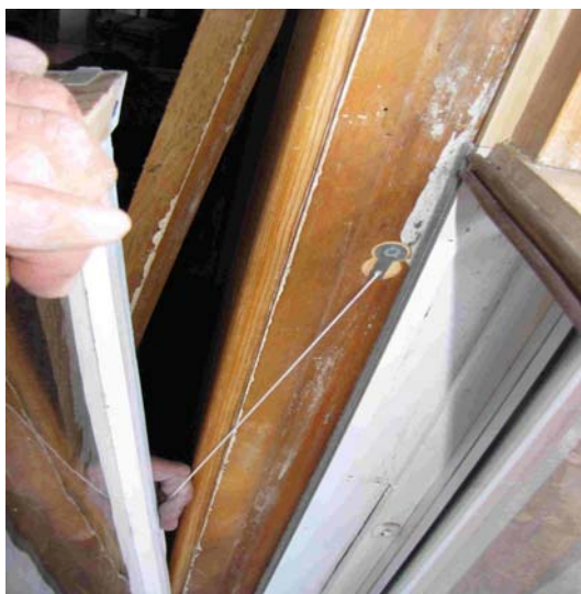
Figure 3-6. Installing spring
