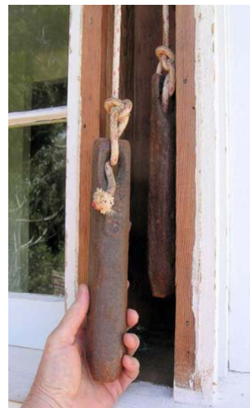
Figure 2-2. Counterweights common to many historic window systems
