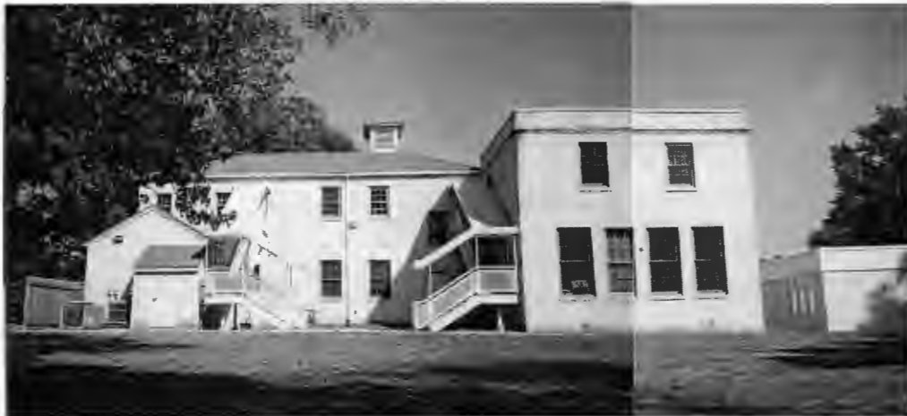
North elevation looking south
