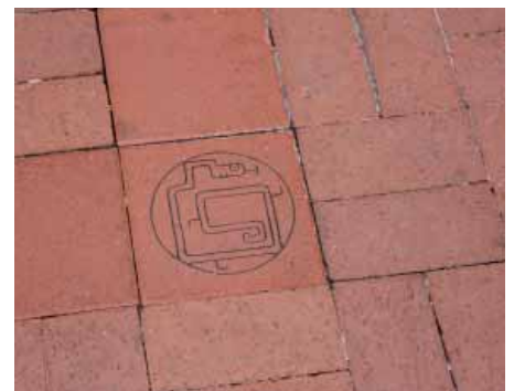
Decorative pavers detail
