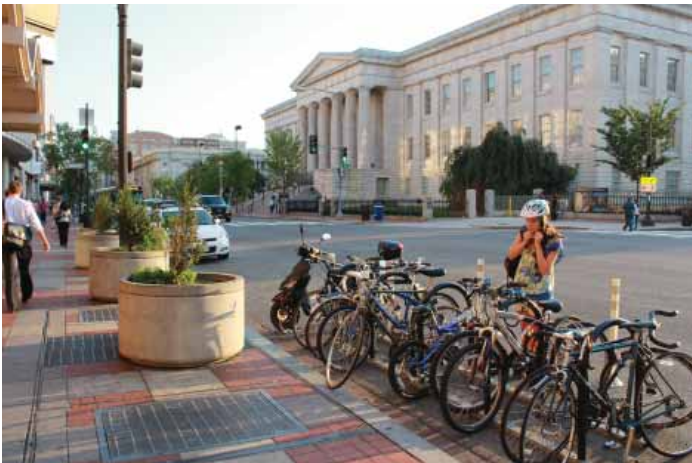
DDOT recently installed on-street bike parking on 7th Street
