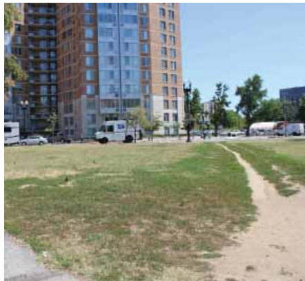
Chinatown Park suffers from poor maintenance
