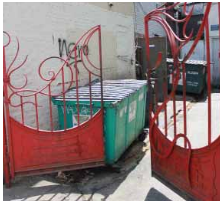
Unscreened foul-smelling alley on H Street
