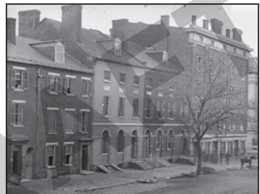
Operable shutters provide shading when needed, improving thermal performance of windows, as well as privacy and storm protection.
