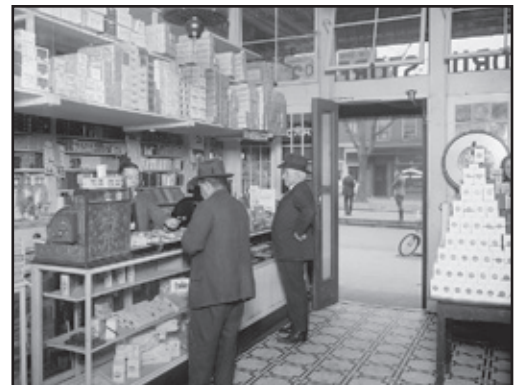
Transoms like the ones on this storefront, improve natural lighting and ventilation on the interior.
