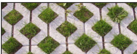
Examples of permeable pavement.
