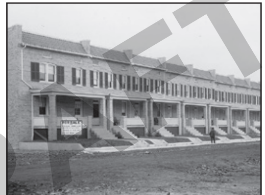
These rowhouses have porches, shutters, and masonry walls, all of which improve performance and energy-efficiency.
