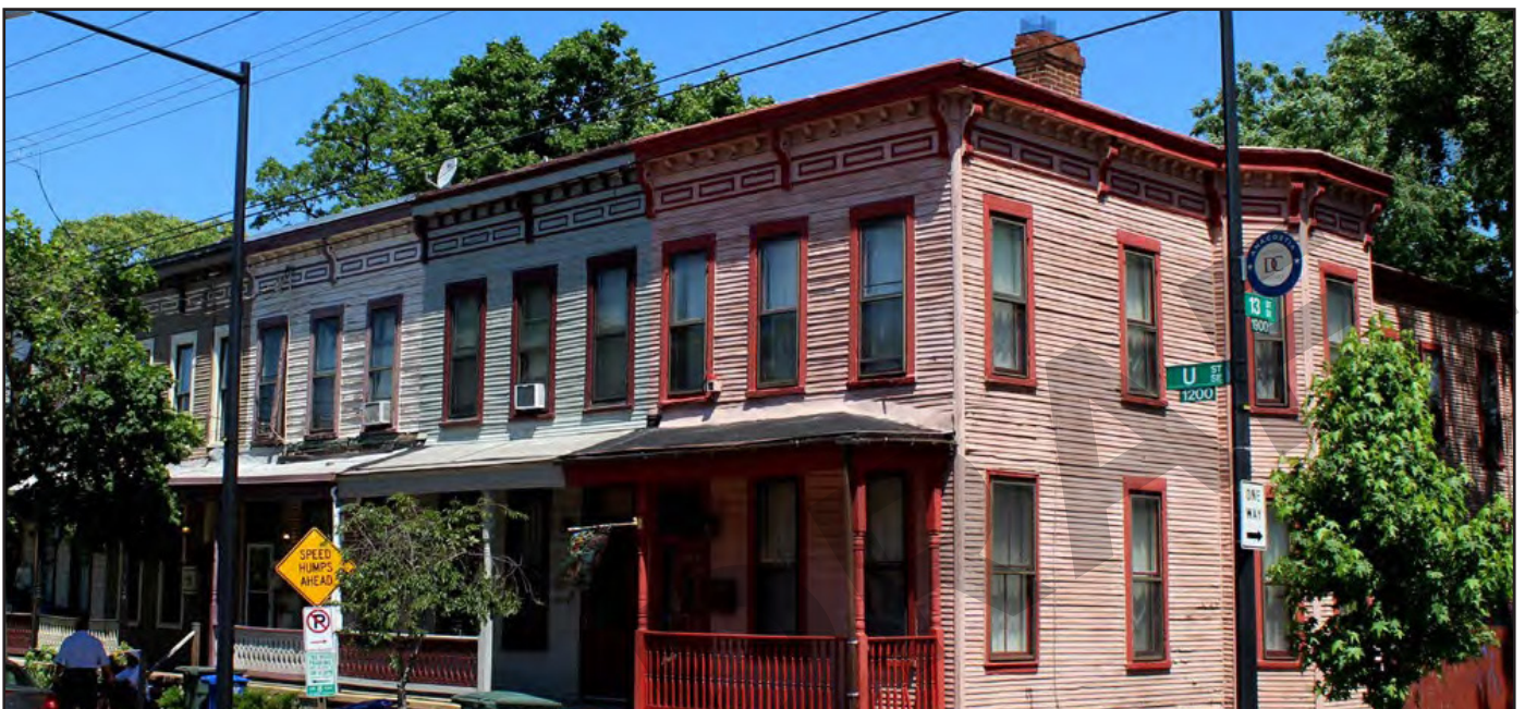
Wood-framed rowhouses in the Anacostia Historic District.
