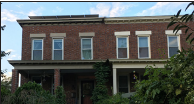
Visibility of solar panels on this corner rowhouse would be significantly improved if they were setback from roof edges.
