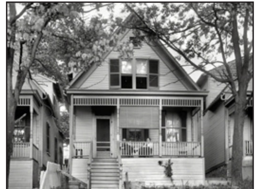
Porches provide sheltered outdoor living space, maximize cross ventilation, and shade exterior walls and windows.
