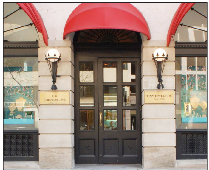
This opening had narrow double doors which did not meet egress requirements. The replacement door was designed to retain a symmetrical appearance with a single sidelight.
