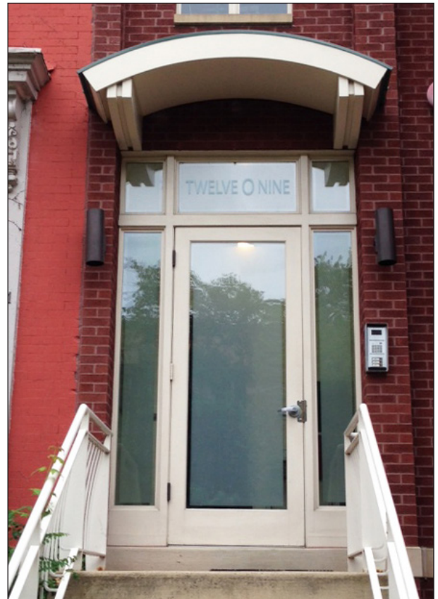
The door on this new building is compatible with the proportions and character of surrounding historic buildings.
