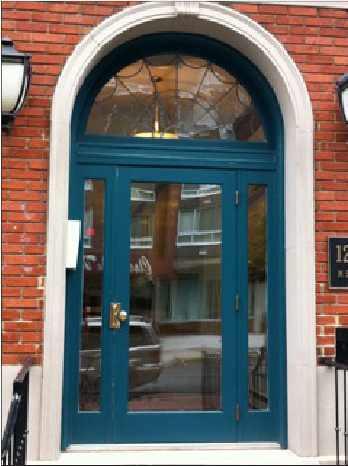
The original narrow double doors on this apartment building were missing and a single wider door was required to meet code requirements. The replacement replicates the symmetrical composition of the original.
