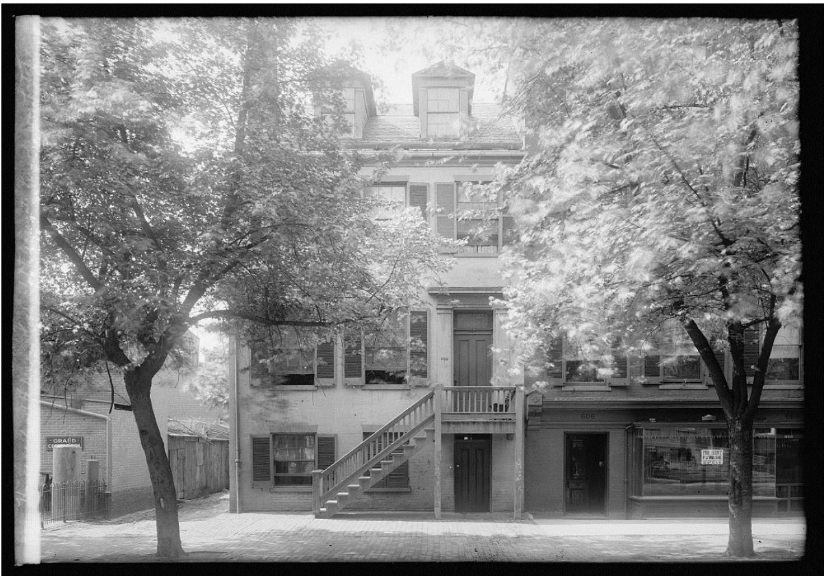
Photo c. 1910-20 of 606 H Street showing conversion of basement level to retail storefront.
