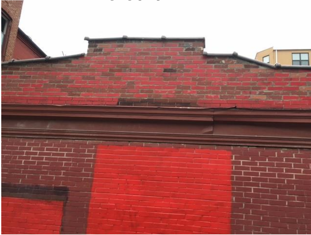
Photos of garage parapet – 501 (rear) H Street, NW
