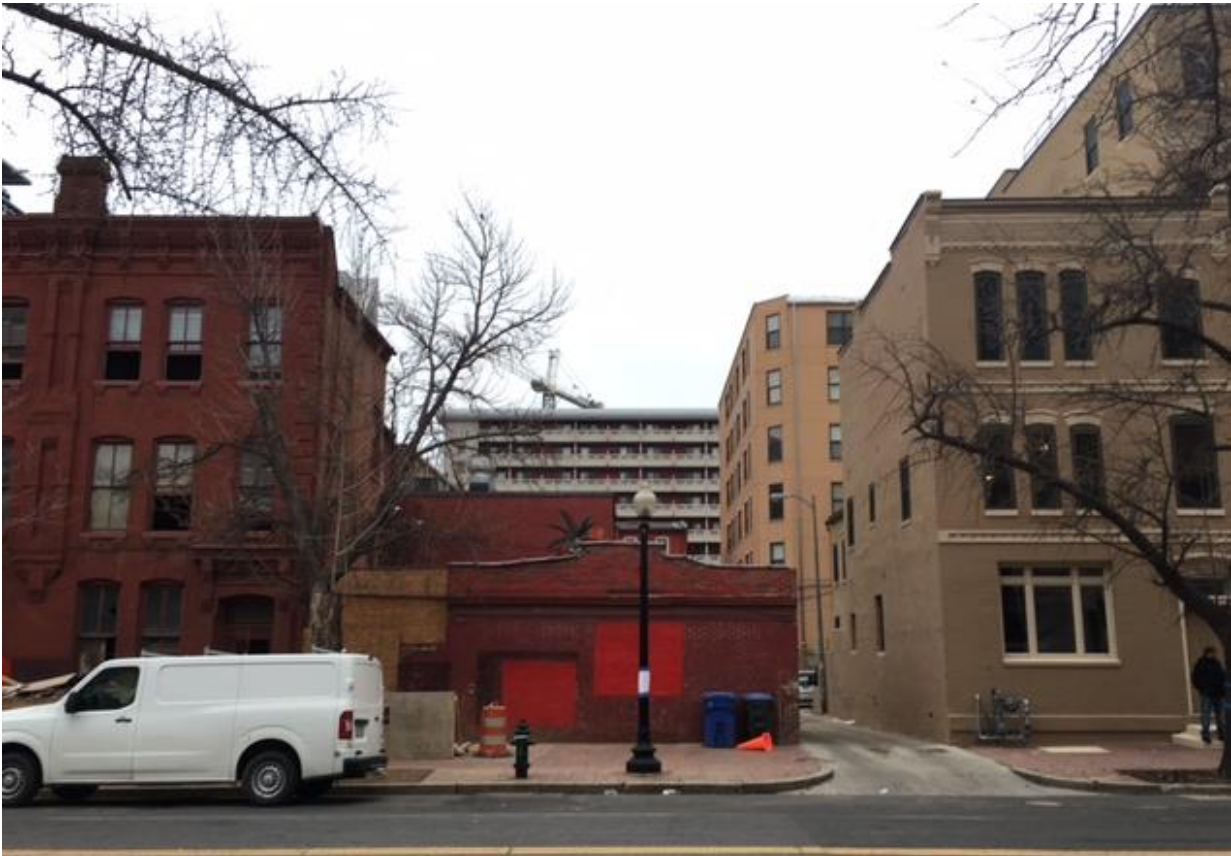
501 H Street, NW and garage: 5 th Street elevation
