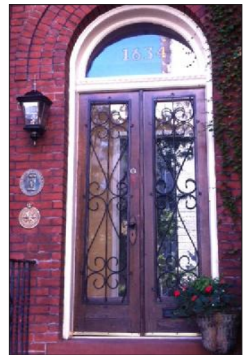
The security gate on the left obscures the building's door. The security bars on the right are integrated into the wood doors, rather than covering them.
