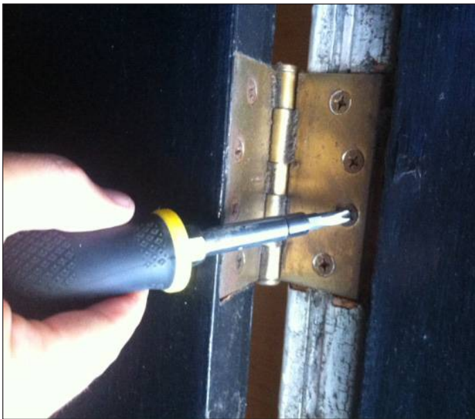
Tightening or replacing hinge screws can fix a door that isn't opening and closing properly.
