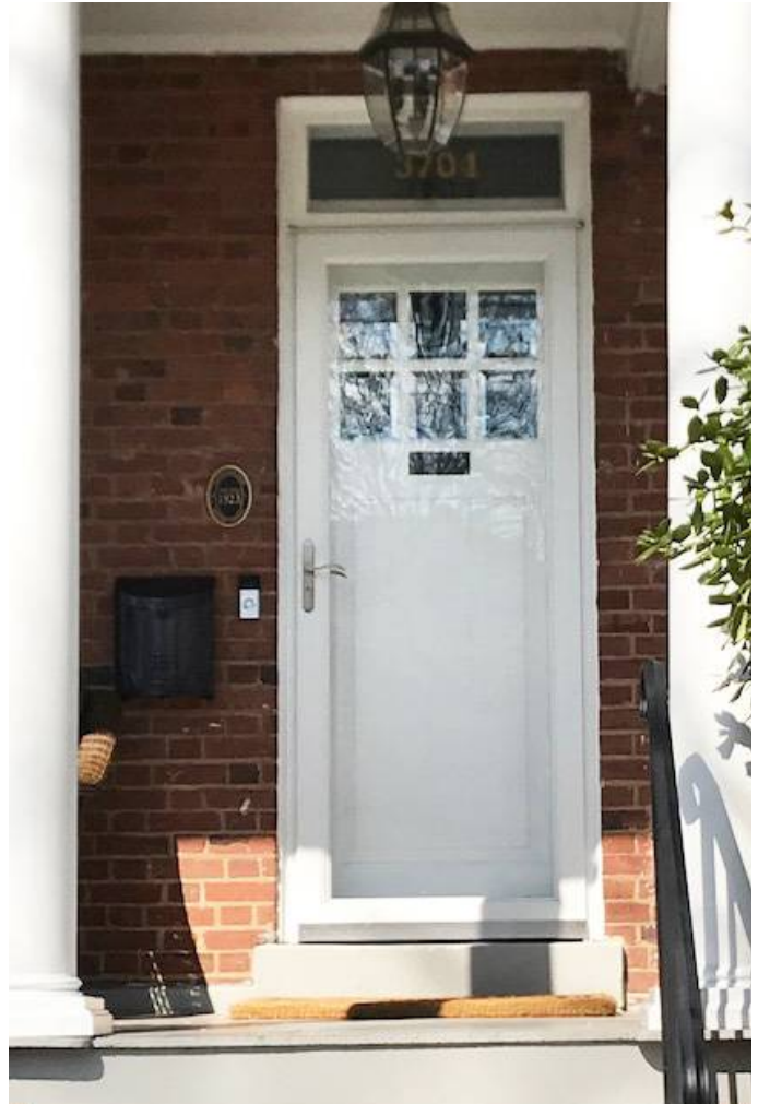
This storm door has narrow stiles and rails and a single pane of clear glass to allow the door to remain visually prominent.
