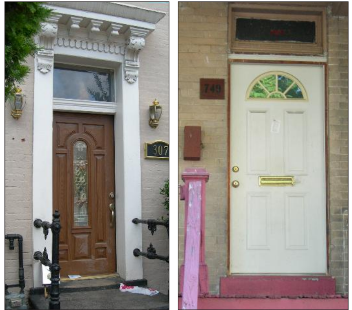
The unusual panel configuration and faux-leaded glazing of the door on the left, and the fanlight glazing in the door on the right have no historical precedent and are not compatible replacements for historic properties.
