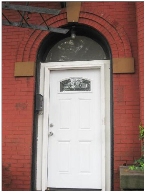
This replacement door is not compatible with the character of the building and not properly sized to fit the opening.
