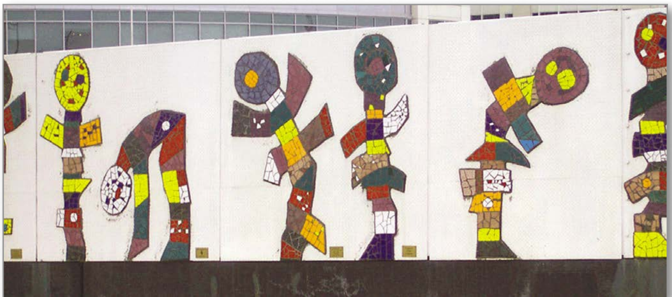
H Street overpass, a.k.a., the "Hopscotch Bridge"
