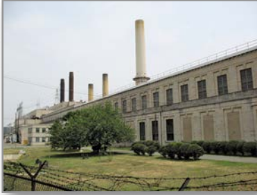
Pepco's oil-powered plant at Benning Road
