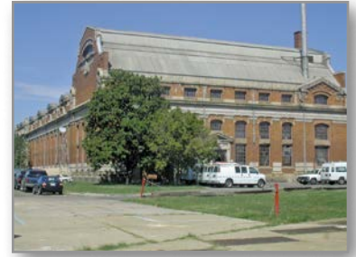
Water and Sewer Authority Building adjacent to the Southeast Federal Center
