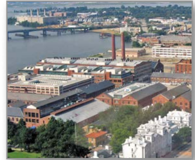
Aerial view of the Navy Yard area
