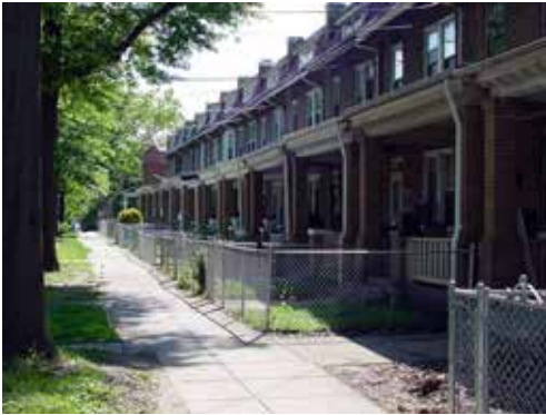
Fence at property line
