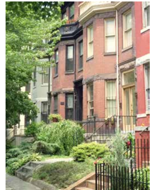
Bay windows promote healthy living by allowing more air and light into building interiors.
