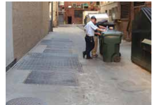
Vaults with grated tops are preferably located in alleys.
