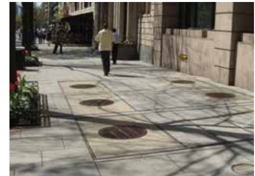
Vaults located in the pedestrian pathway are required to have solid covers that match the adjacent sidewalk.
