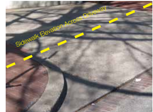
The elevation of the sidewalk where it crosses the driveway should be level with the adjacent sidewalk.
