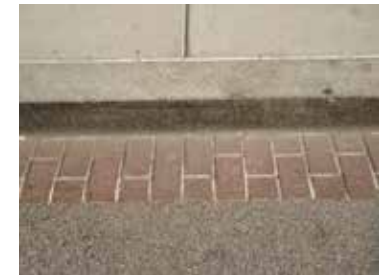
Granite curb with brick gutter
