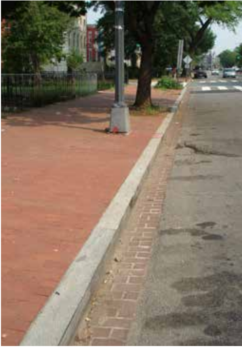
Curbs and gutters define the boundary between the roadway and the sidewalk.
