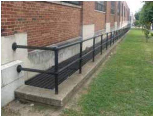
Areaways are used to get light into lower levels of buildings.
