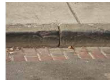
Bluestone curb with brick gutter
