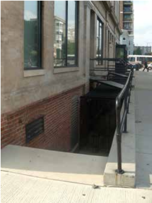
Areaways may be used for steps providing secondary building access to lower levels.
