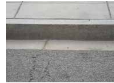
Granite curb with concrete gutter
