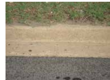
Concrete curb with concrete gutter
