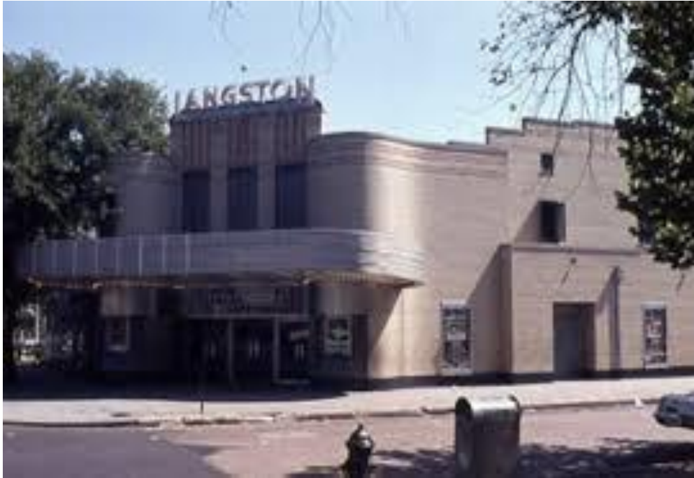
Image 11: Langston Theater at 25 th Street and Benning Road NE, built 1945, razed in the 1970s (Historical Society of Washington).
