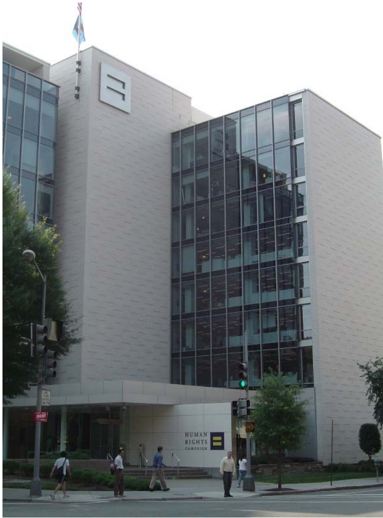
Figure 17: B'nai B'rith International Headquarters (1957) at 1640 Rhode Island Avenue, NW, by Corning & Moore. (Robinson & Associates, 2008)
