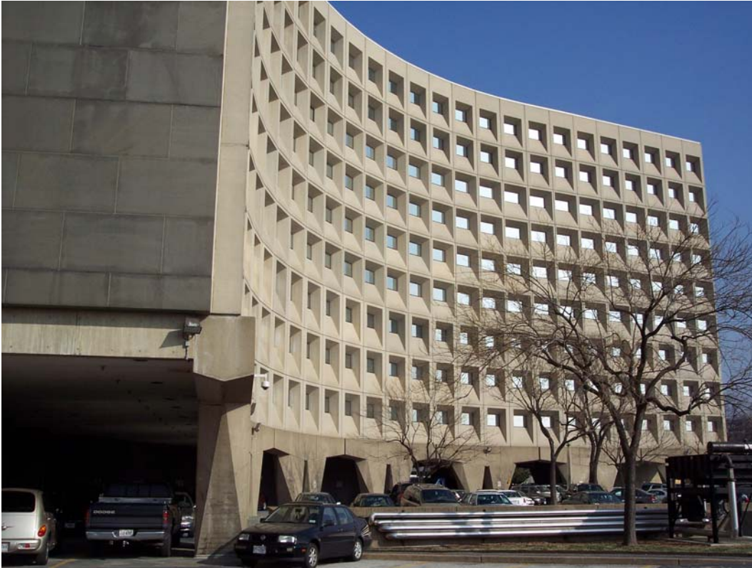
Figure 66: The U.S. Department of Housing and Urban Development (HUD) (1965-68) at 451 Seventh Street, SW, by Marcel Breuer. (Robinson & Associates, 2008)
