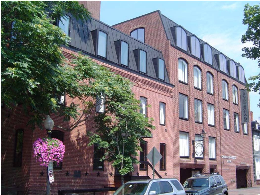
Figure 49: Canal Square designed by Arthur Cotton Moore/Associates in 1970. (Robinson & Associates, 2008)
