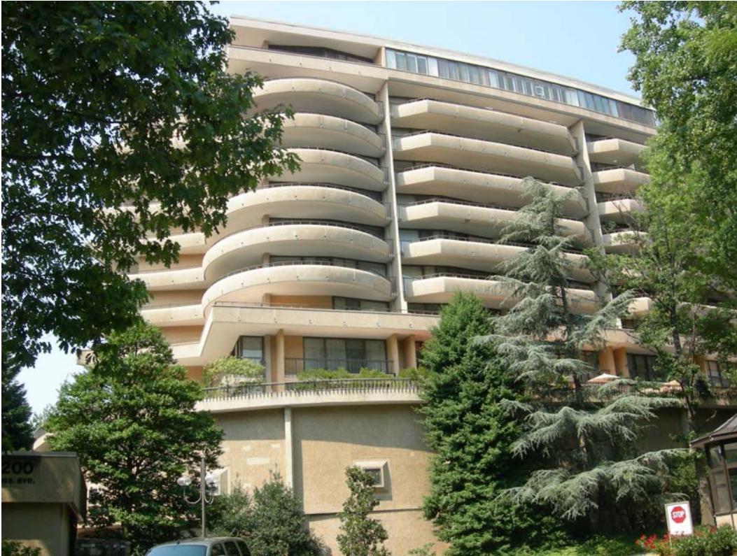
Figure 48: Foxhall Apartments (1970-76) at 4200 Massachusetts Avenue, NW, by Fischer and Elmore. (Robinson & Associates, 2008)
