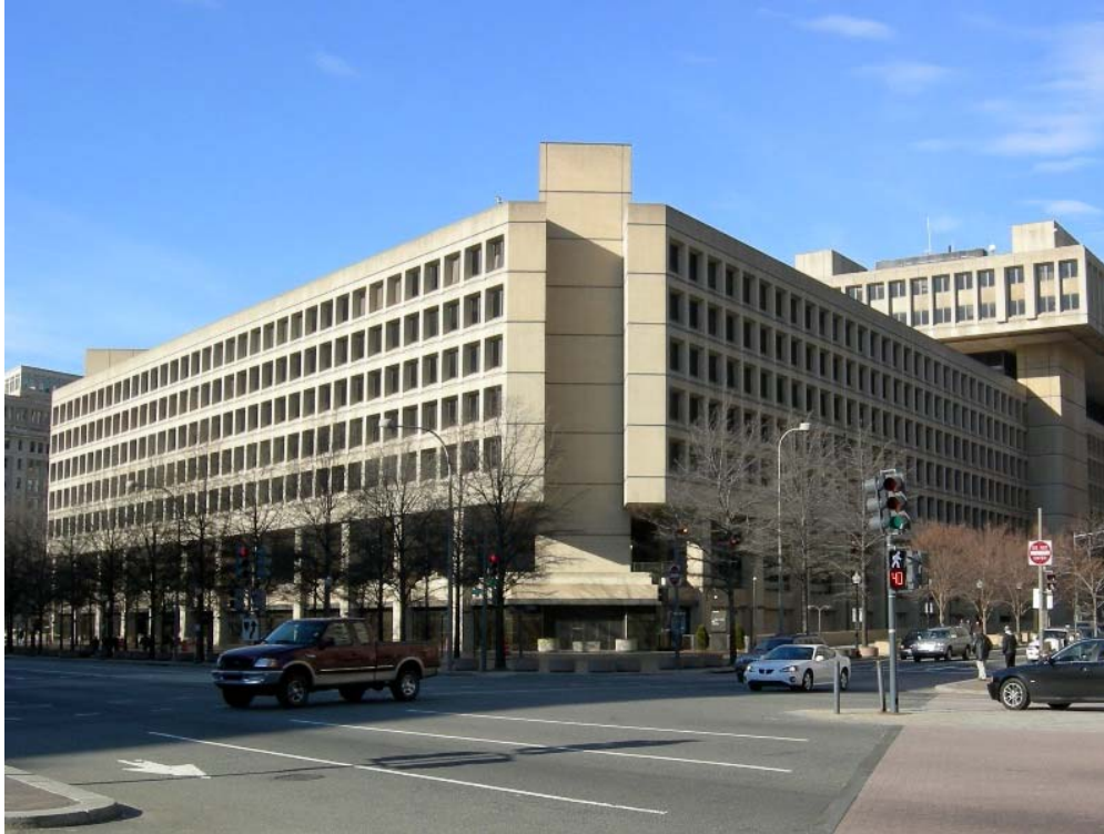
Figure 23: The FBI Building (1967-72), located along Pennsylvania Avenue between 9th and 10th streets, NW, designed by C.F. Murphy & Company with Stanley Gladych as principal designer. (Robinson & Associates, 2006)
