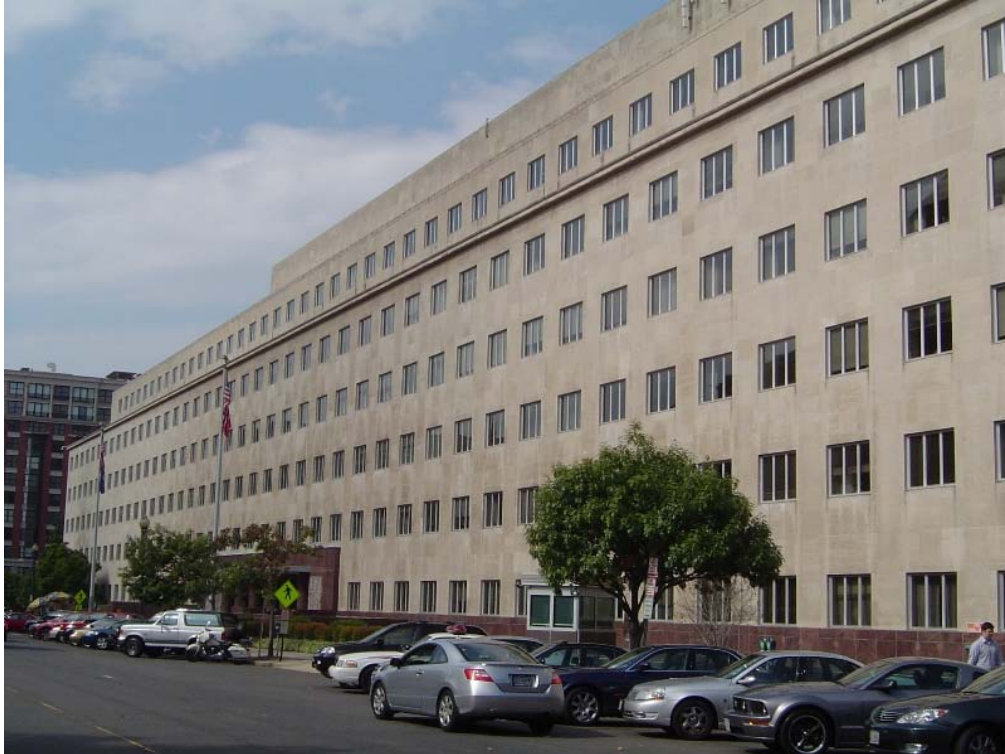
Figure 8: The General Accounting Office (1949-51) by Gilbert Stanley Underwood was the first federal office building in Washington to rely entirely on florescent lights rather than light courts or skylights to illuminate interior office space. (Robinson & Associates, 2008)
