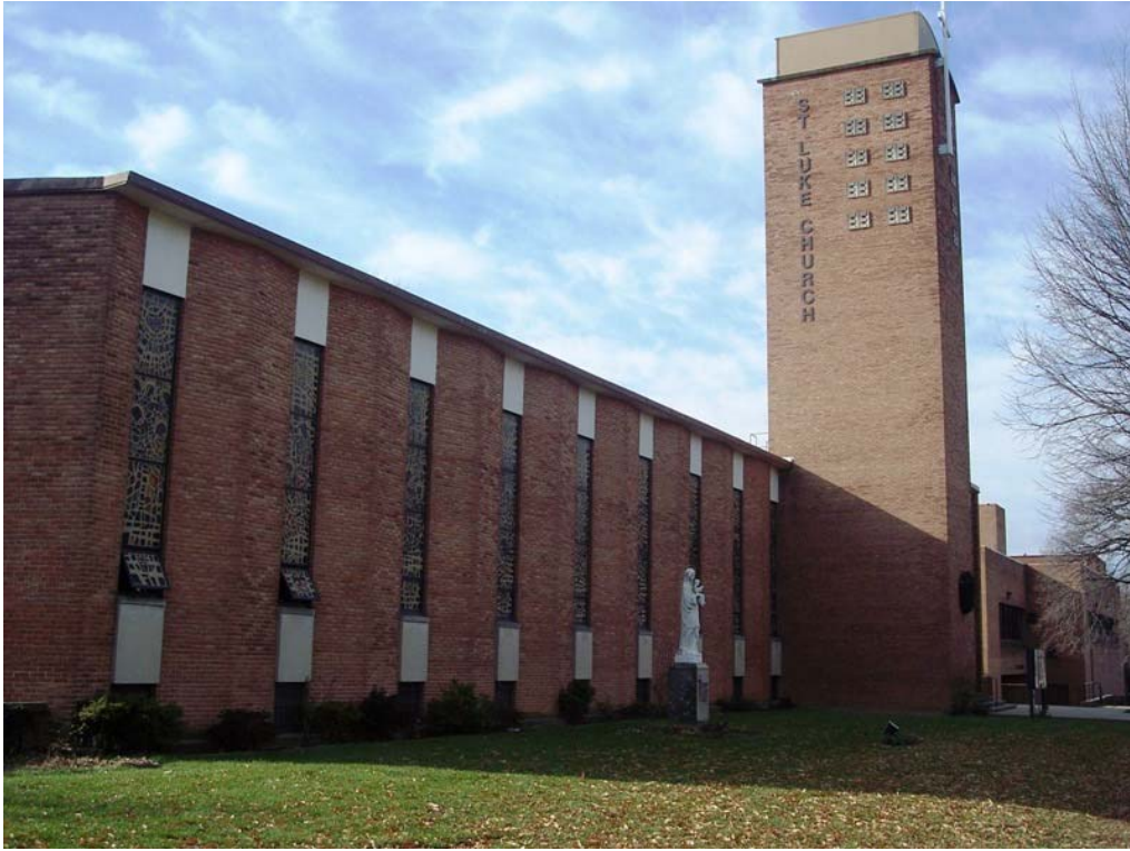
Figure 18: St. Luke's Church (1957) at 4925 East Capitol Street, SE, by Thomas E. Locraft & Associates. (Robinson & Associates, 2006)
