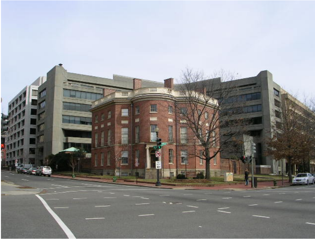
Figure 60: AIA Headquarters (1972-74) at 1735 New York Avenue, NW, by The Architects Collaborative (TAC). (Robinson & Associates, 2008)
