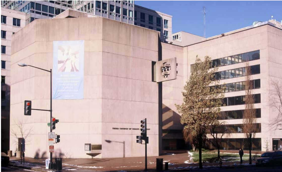
Figure 57: The Third Church of Christ, Scientist and the Christian Science Monitor office building (1971) at 16th and I streets, NW, by Araldo Cossuta of I.M. Pei Associates. (Photo courtesy Walter Smalling)
