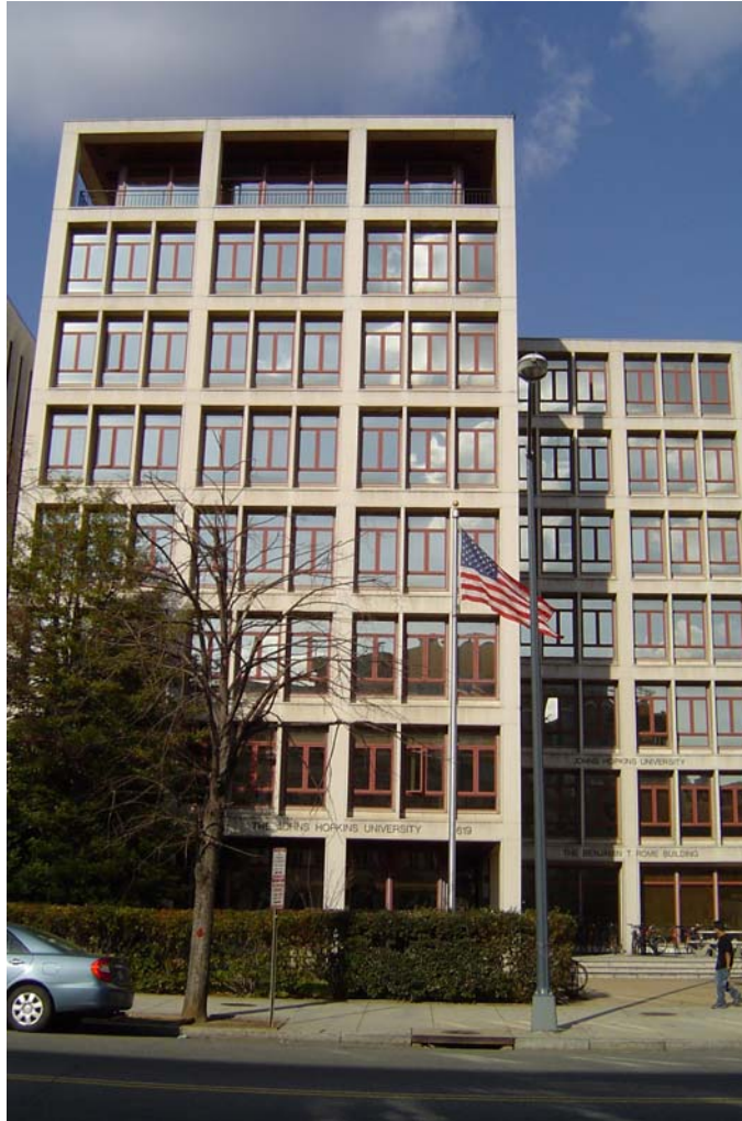
Figure 31: Forest Industries Building (1961) at 1619 Massachusetts Avenue, NW, by Keyes, Lethbridge & Condon. (Robinson & Associates, 2005)
