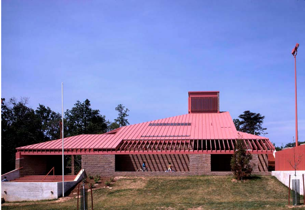
Figure 65: Fairfax Village Recreation Center (1969) at 41st Street and Alabama Avenue, SE, by Hartman-Cox. (Photo courtesy Hartman-Cox)
