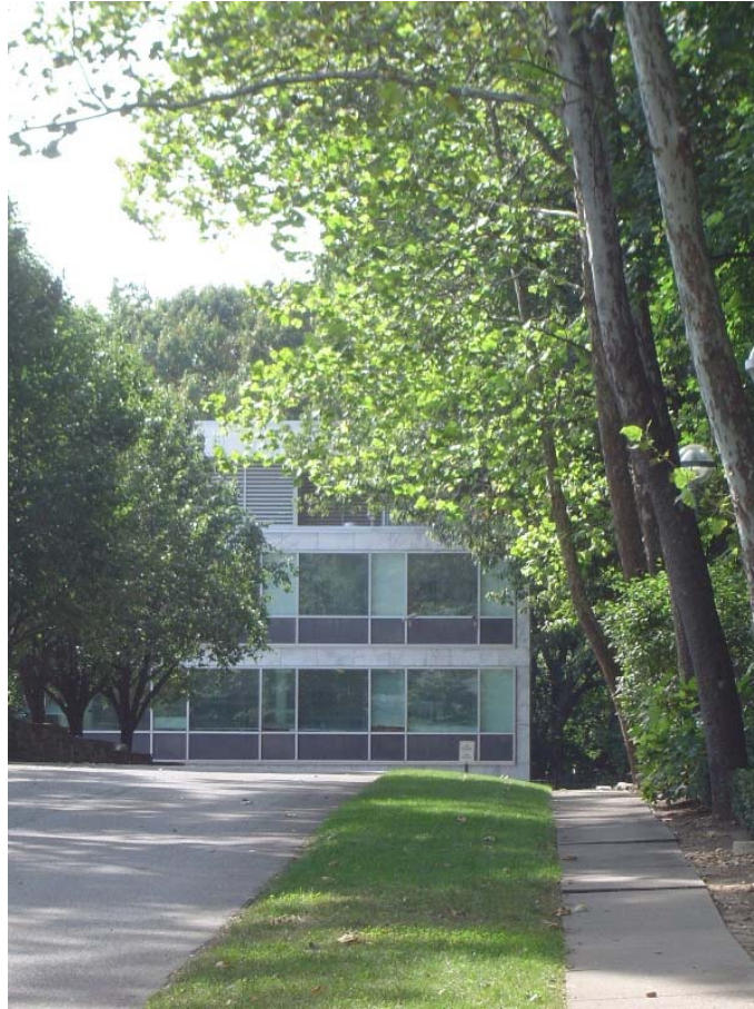
Figure 40: The Embassy of Denmark (1960), designed by Vilhelm Lauritzen. (Robinson & Associates, 2008)
