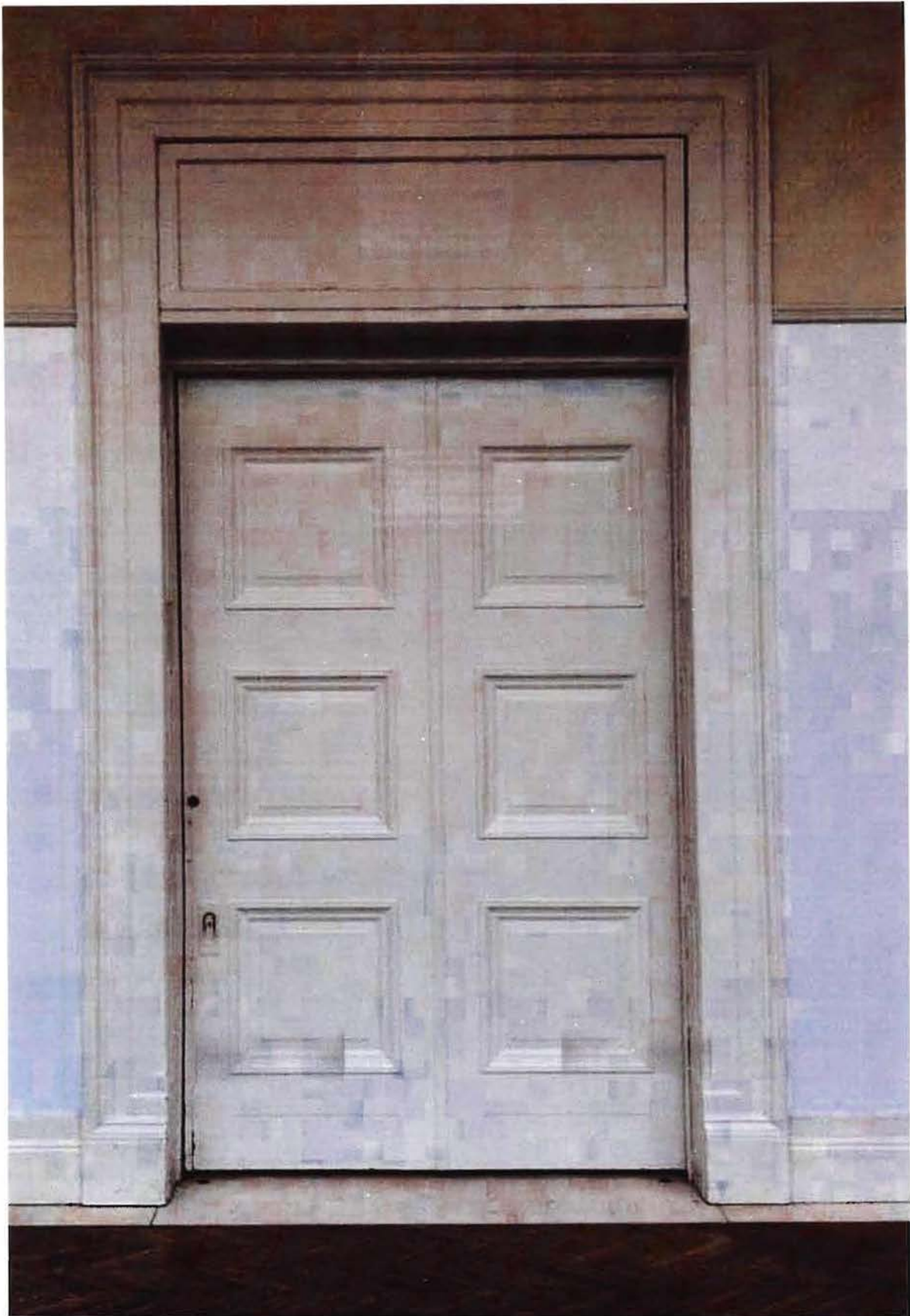
Illustration 22: Detail of Gallery-to-Atrium Pocket Door, With Herringbone Pattern Wooden Floor and Marble Border.
