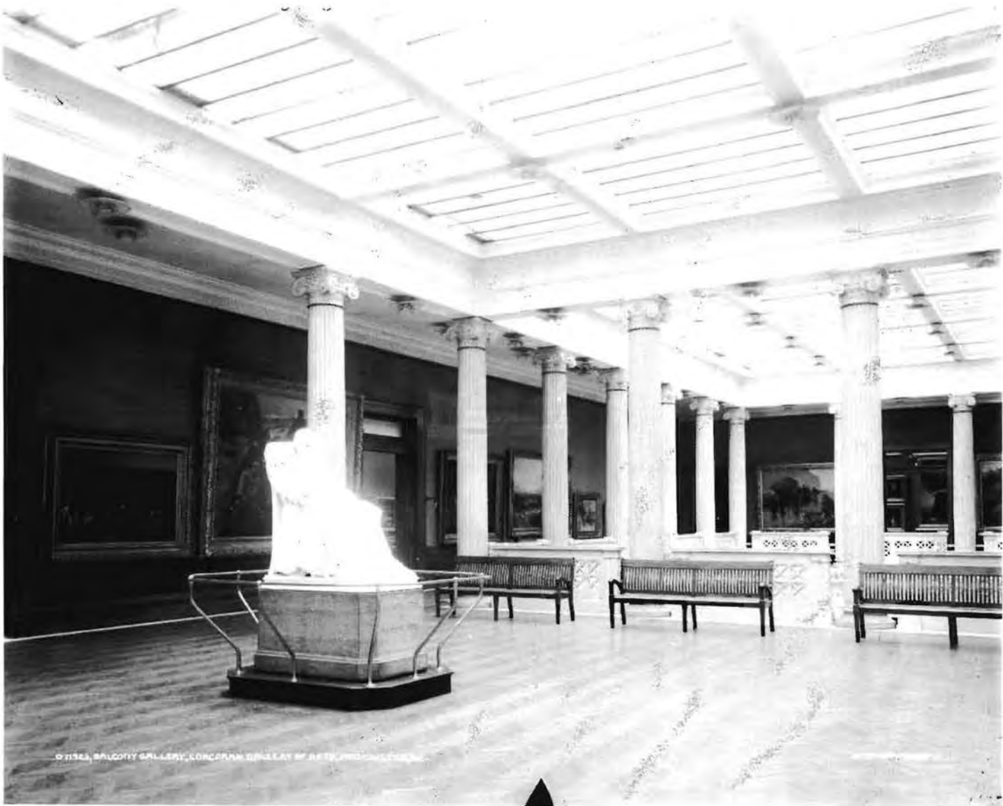
Illustration 14: Balcony, Central Gallery in Historic View
