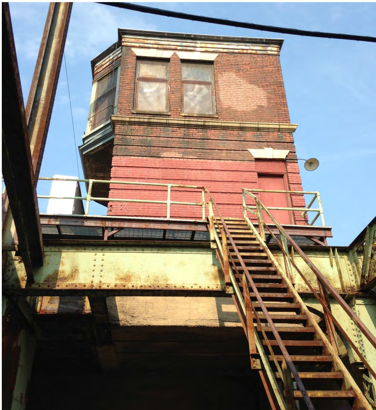
Figure 3. Steel frame staircase with concrete treads attached to steel platform on the East Elevation, CP Virginia Tower.
