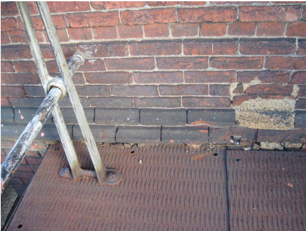
Figure 4. Water table consisting of two rows of red concave plinth bricks, CP Virginia Tower.
