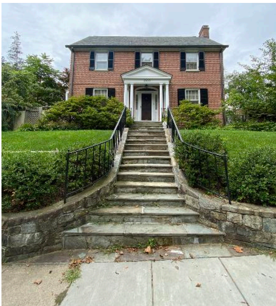
Stone steps, walkway, and retaining wall
