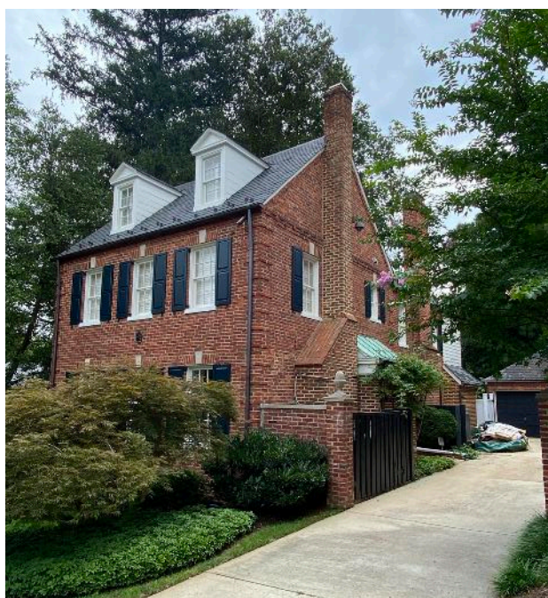
Gabled and hipped roofs with dormers and chimneys
