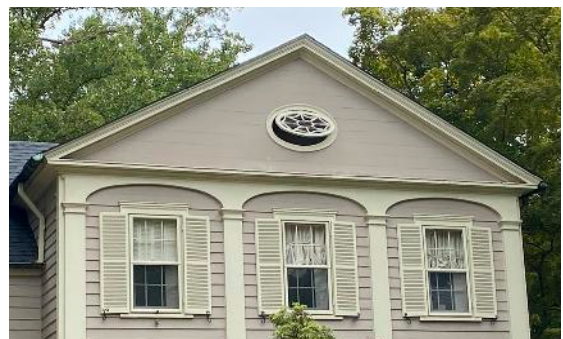
Multi-paned double hung wood windows with shutters are a defining architectural feature of Colony Hill homes.
