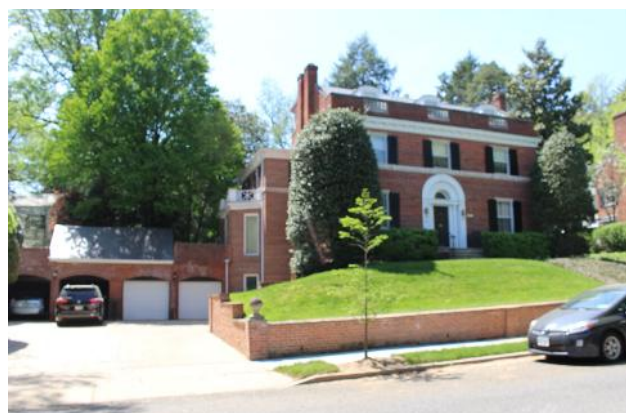
Low exterior masonry site walls
