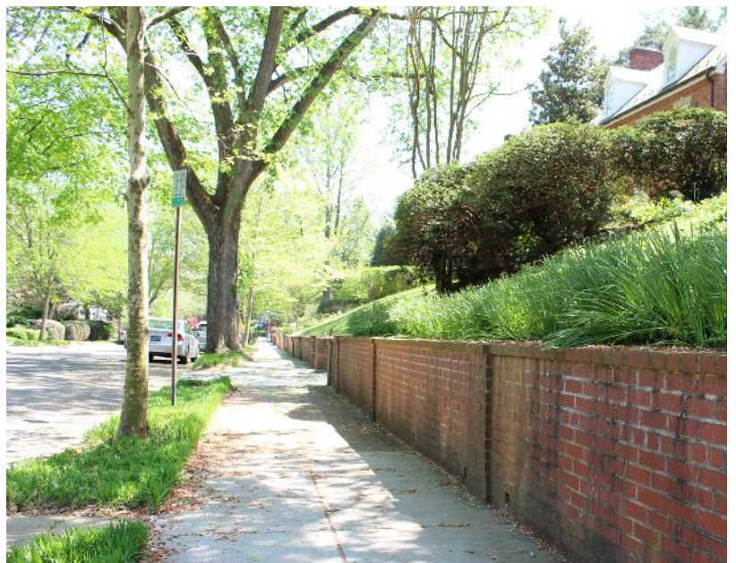
Continuous brick masonry site wall
