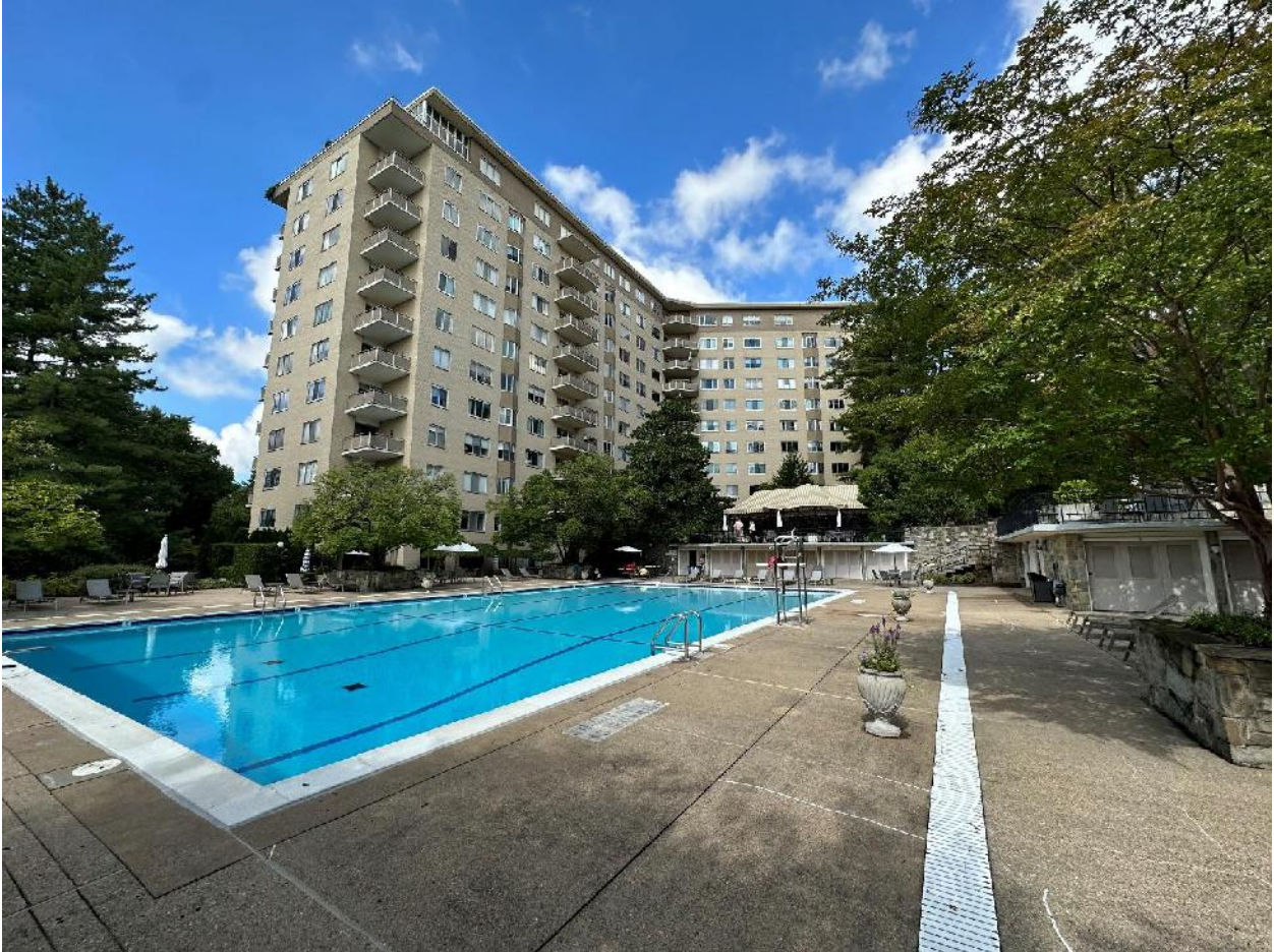
7 of 26. View of pool area from southern pergola.
