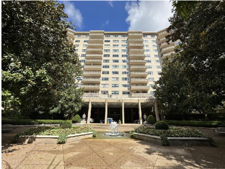
Figure 2. Fountain and courtyard looking north towards the building lobby. Photo by EHT Tracerics.
