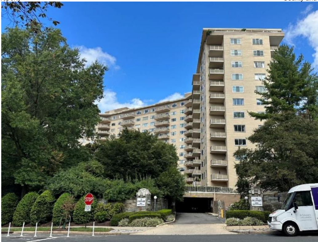
Figure 5: The southern elevation serves as the primary façade. Photo by EHT Tracerics.
