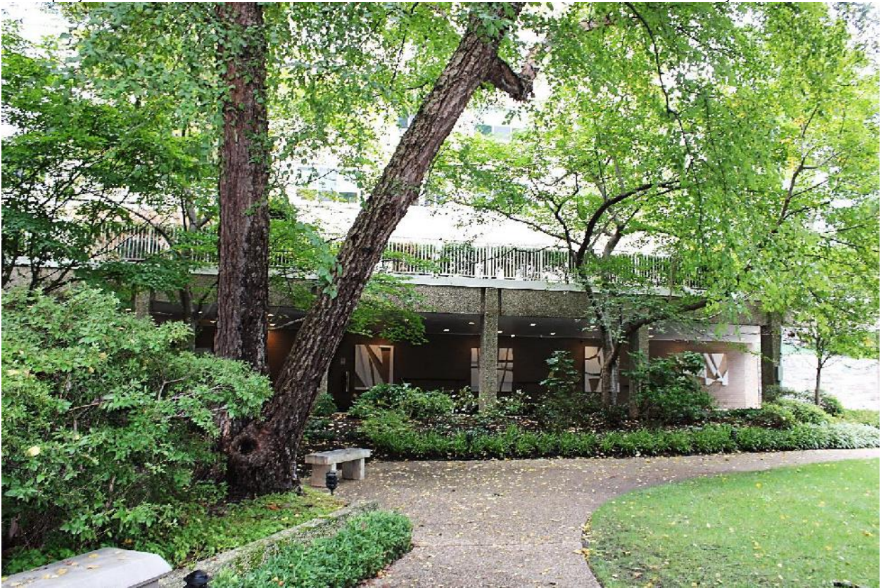
9 of 26. Single-story colonnade with terrace roof, southeastern wing in distance.
