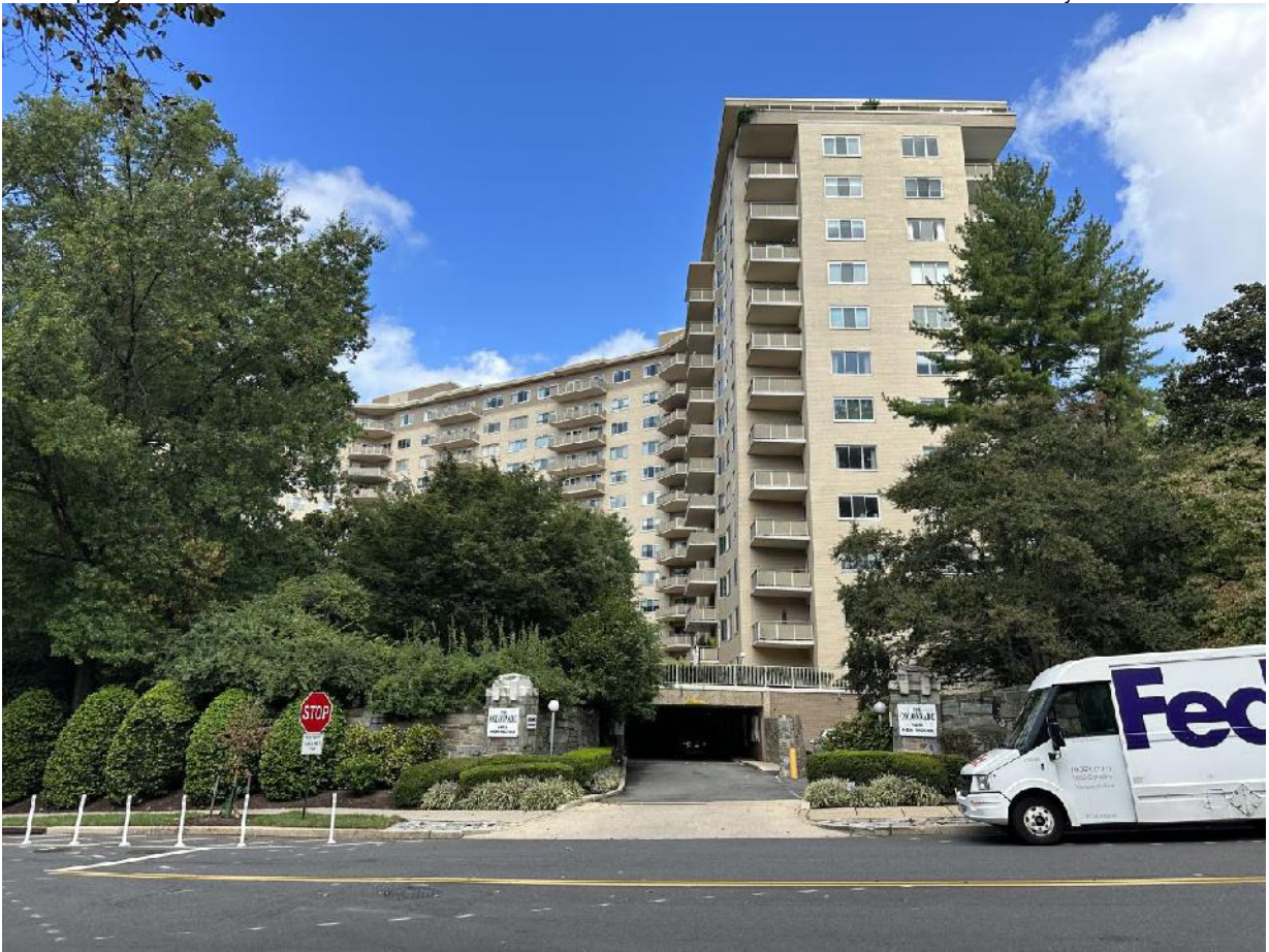
1 of 26. View of building and covered driveway entry from Tunlaw Road.
