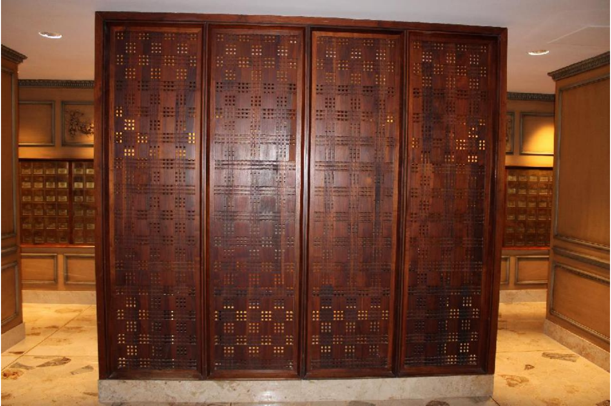
24 of 26. View of original decorative screen wall.
