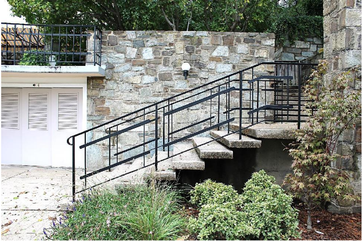
11 of 26. Pool area with cabana entry, original metal railings, cantilevered stone steps, and stone retaining walls. Cabana and pool's second level visible.
