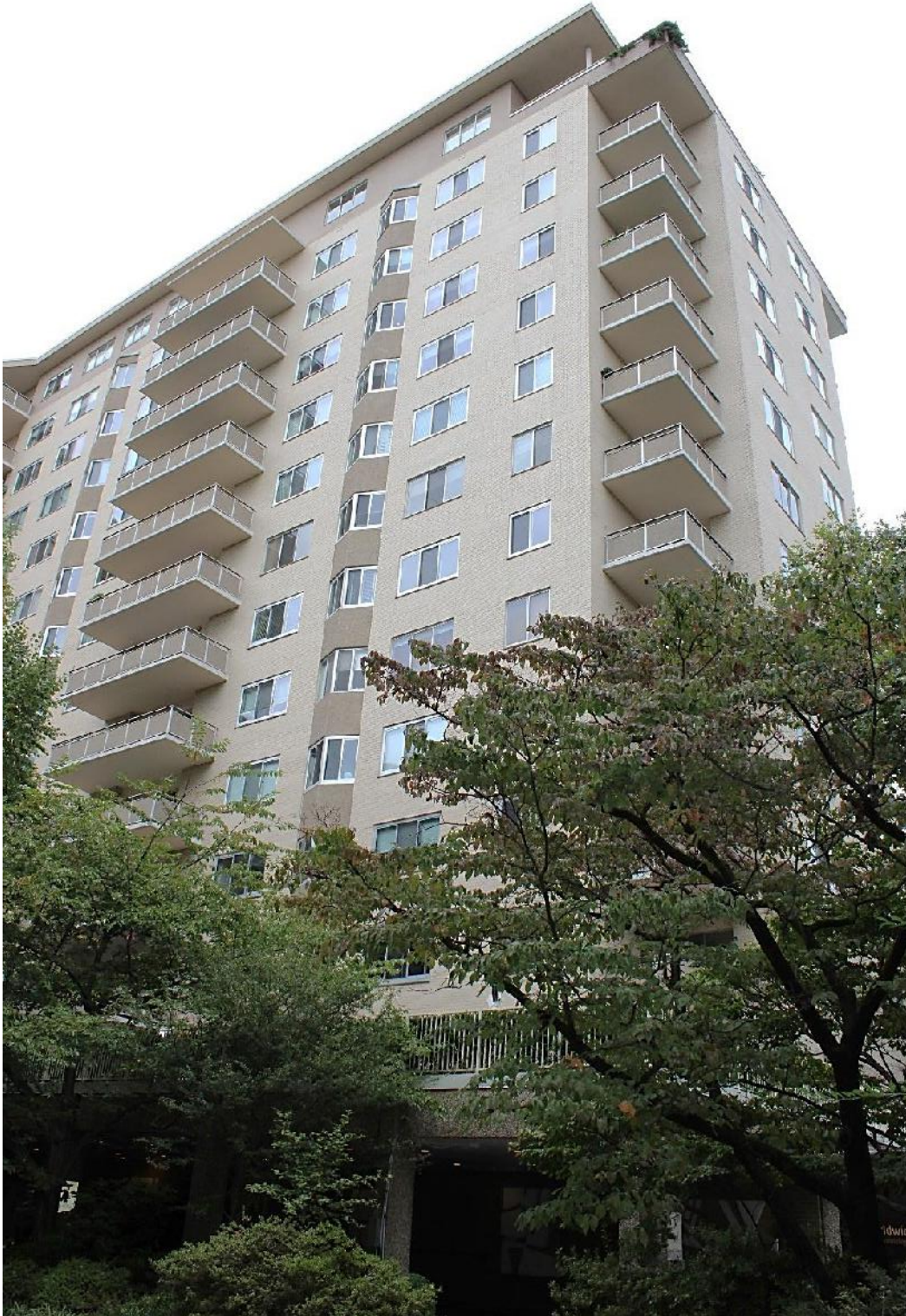
2 of 26. View of building from courtyard.
