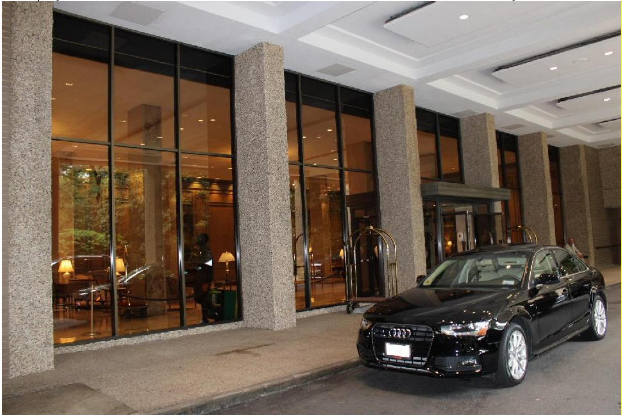
10 of 26. View of lobby from two-story colonnade.
