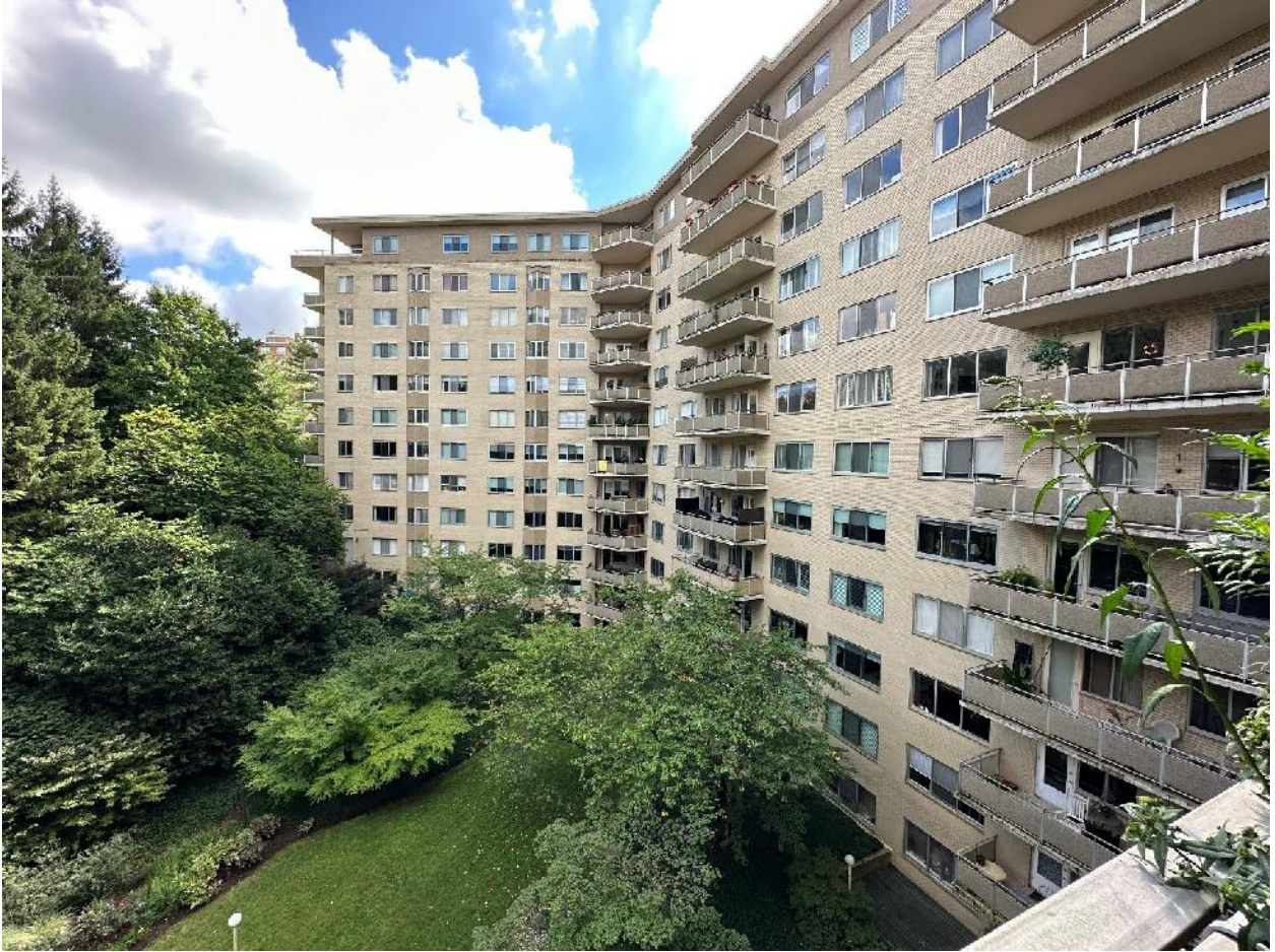
6 of 26. View of south courtyard and rear of building from balcony.
