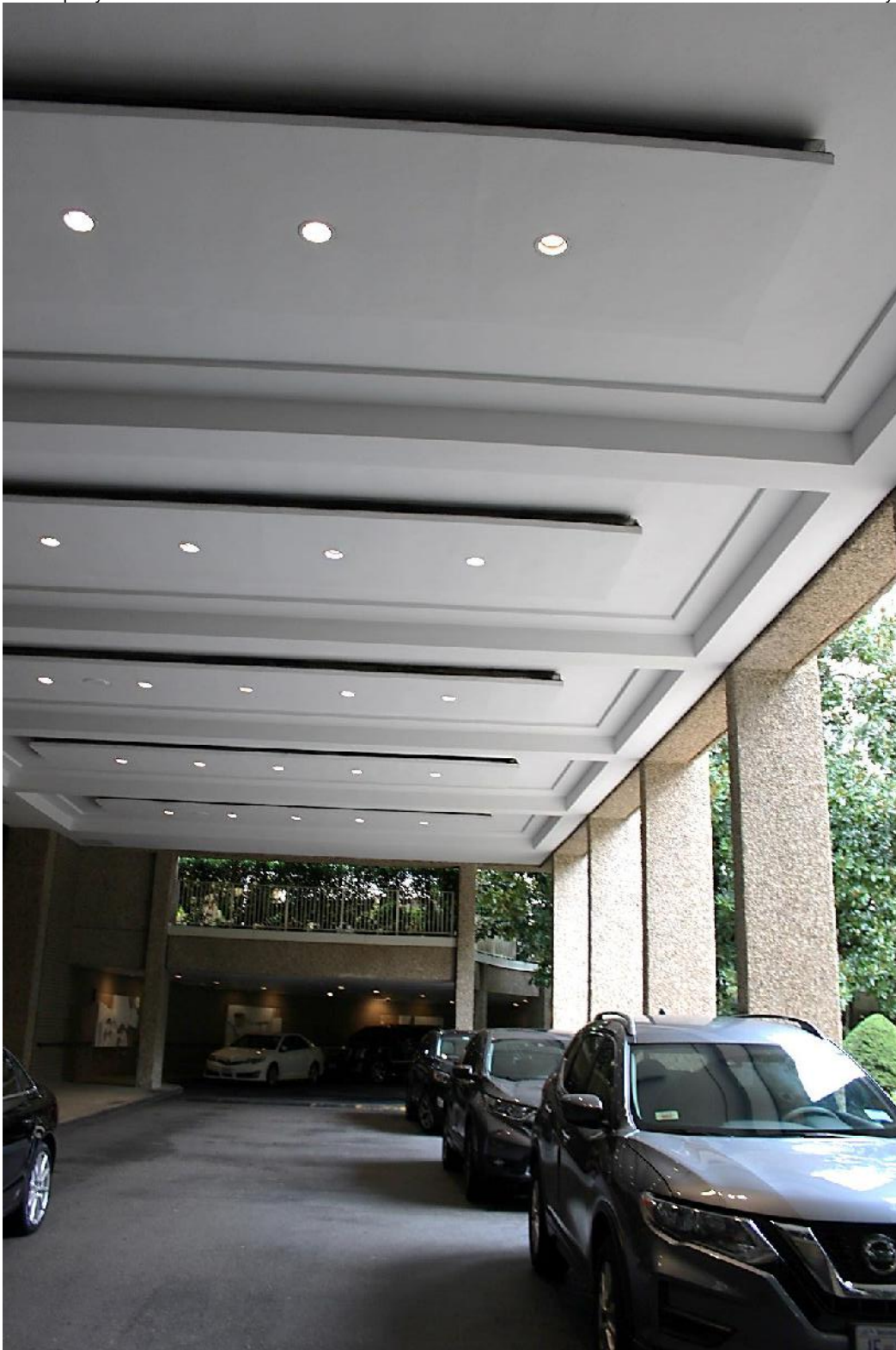
8 of 26. Two-story colonnade.
