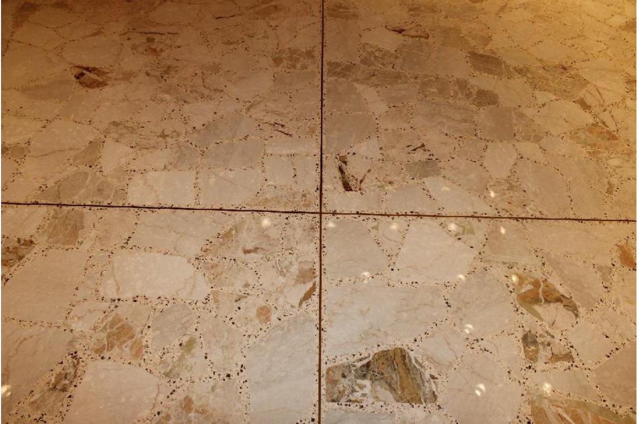
25 of 26. Detail of terrazzo floors with inlaid marble.
