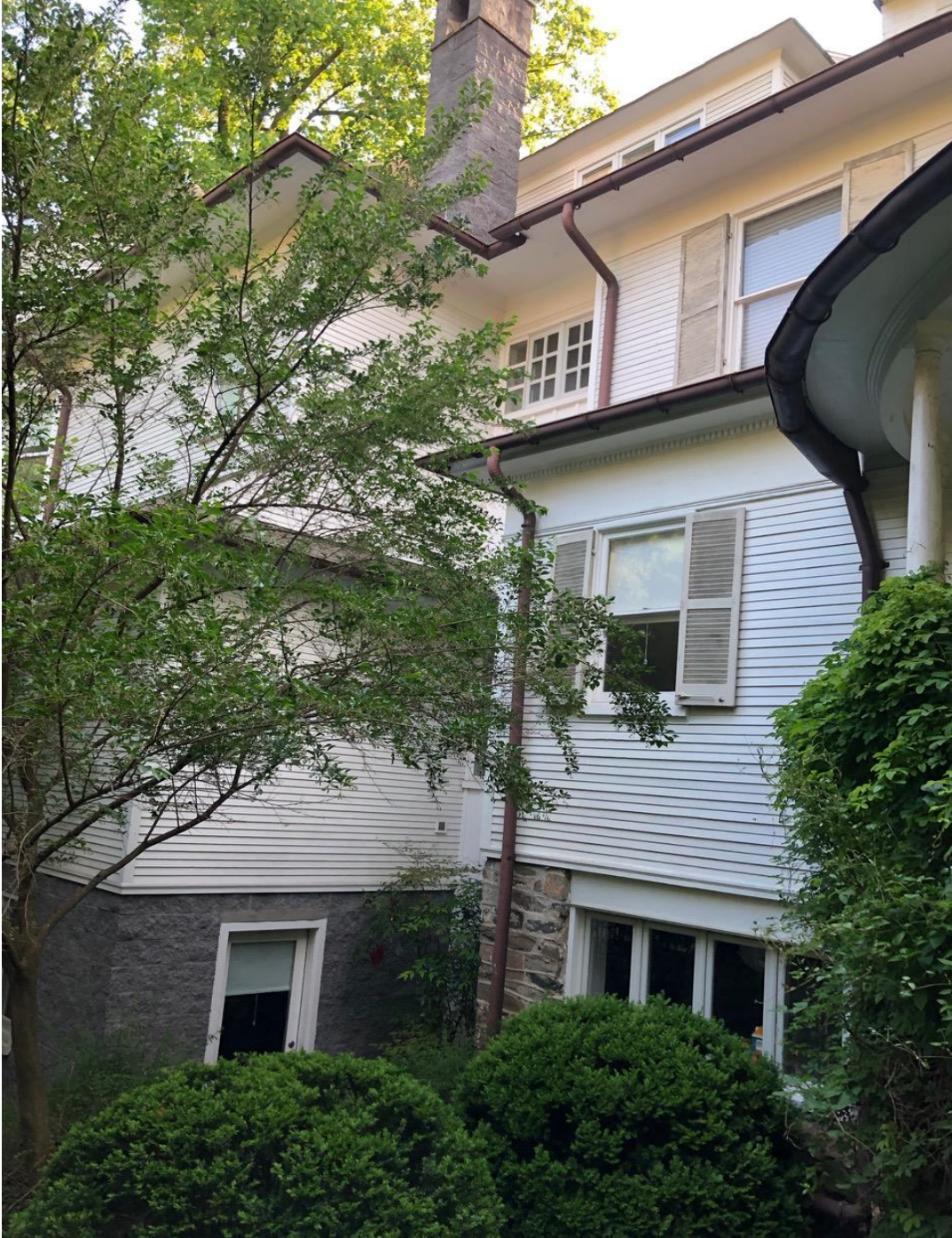
This rear addition in Cleveland Park projects past the side wall of the original house using a recessed hyphen to differentiate between the two.
