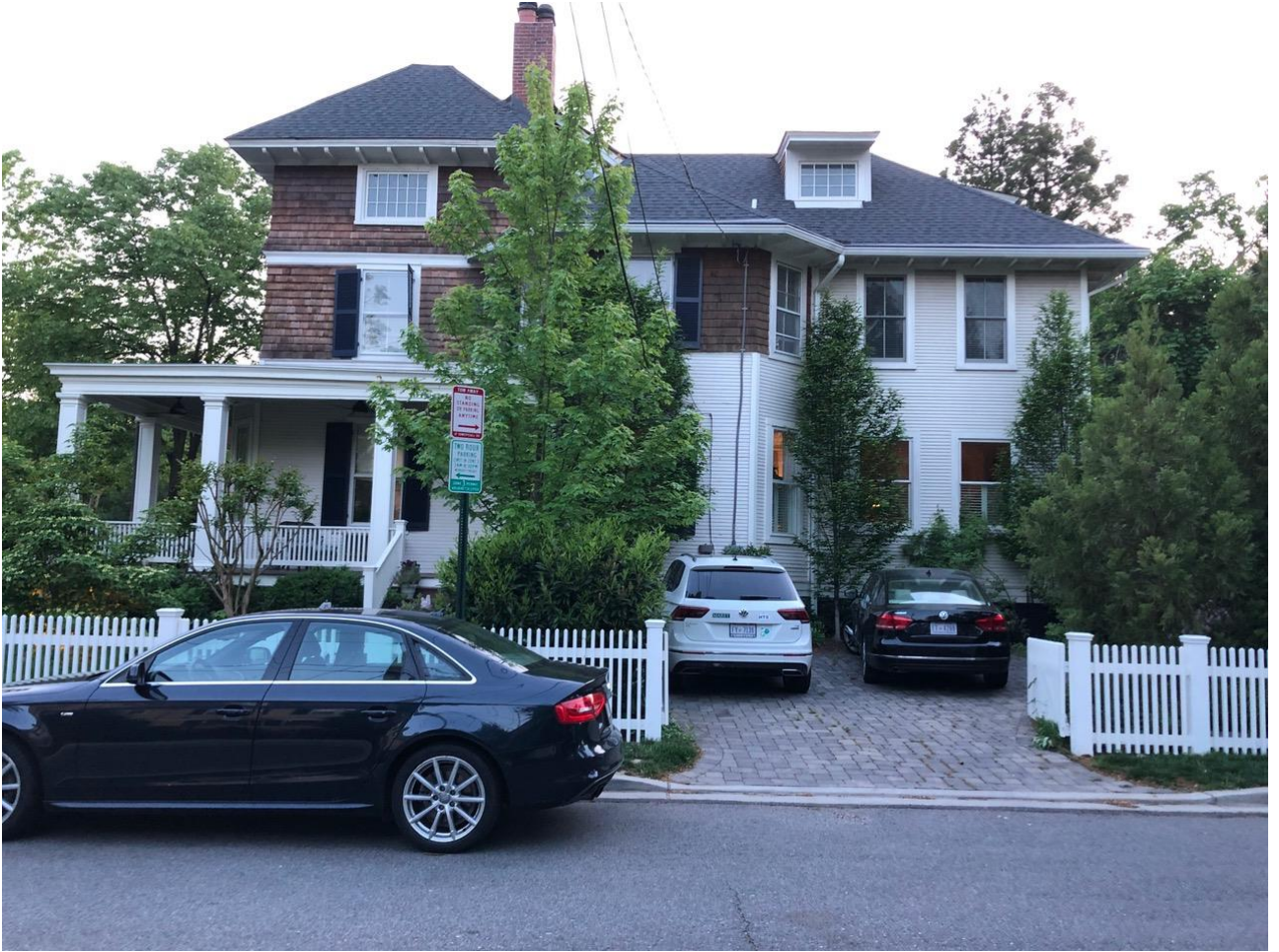
This rear addition on a corner house in Cleveland Park is pulled back from the plane of the original side elevation to achieve a subordinate relationship to the house.
