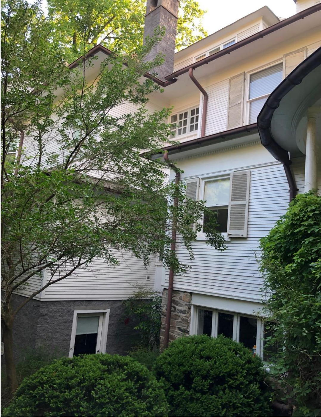
This rear addition in Cleveland Park projects past the side wall of the original house using a recessed hyphen to differentiate between the two.
