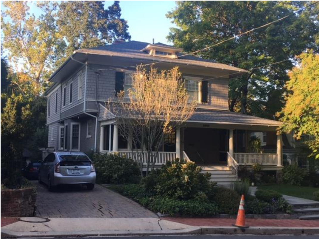
3215 from sidewalk in front of 3216 Newark
