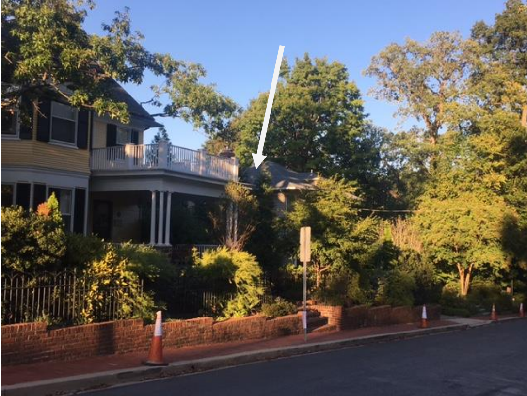
View of west roof slope of 3215 Newark from sidewalk in front of 3300 Newark
