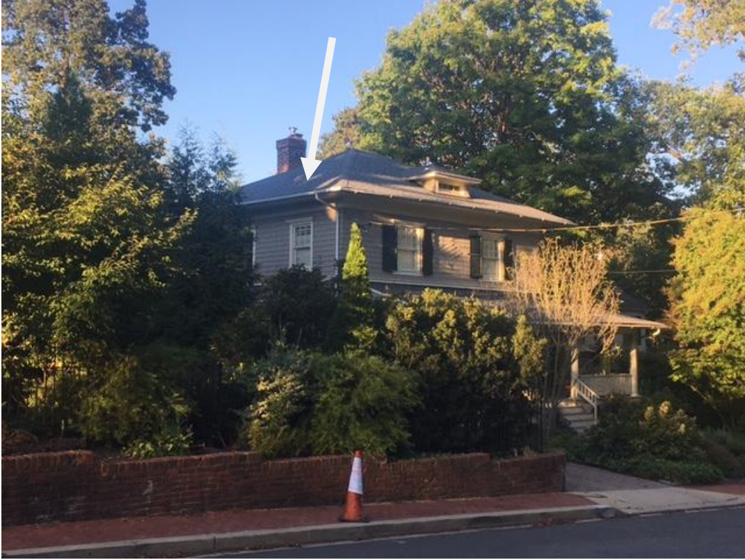
3215 from sidewalk in front of 3218 Newark
