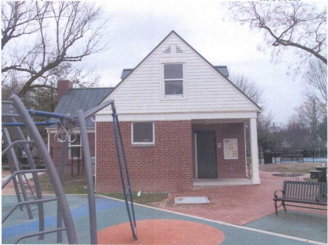
Chevy Chase Playground and Field House Washington, DC March 20, 2016 Kent Boese Chevy Chase Field House, Northwest Elevation 10/15
