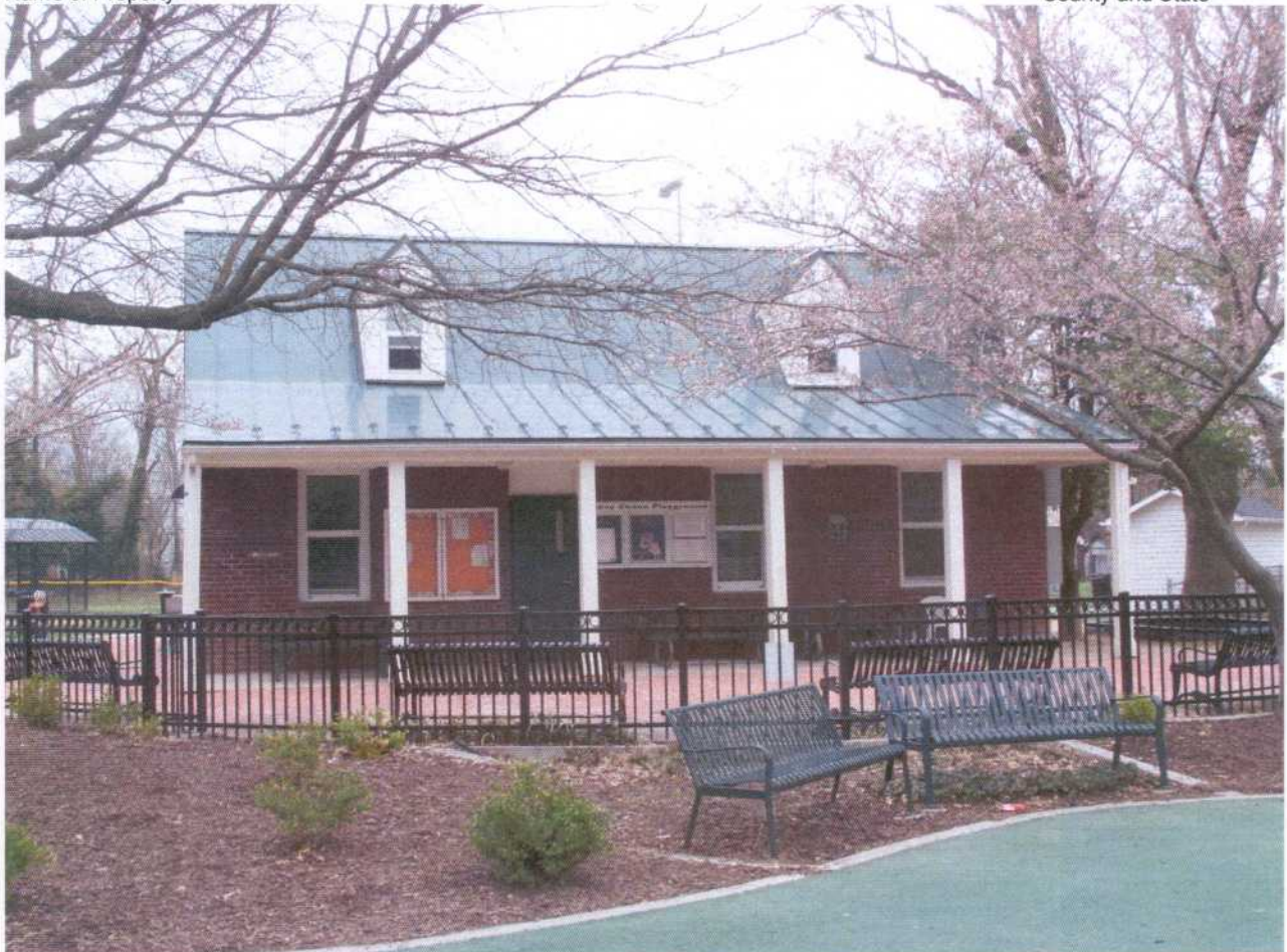
Chevy Chase Playground and Field House Washington, DC March 20, 2016 Kent Boese Chevy Chase Field House, Southeast Elevation 7/15
