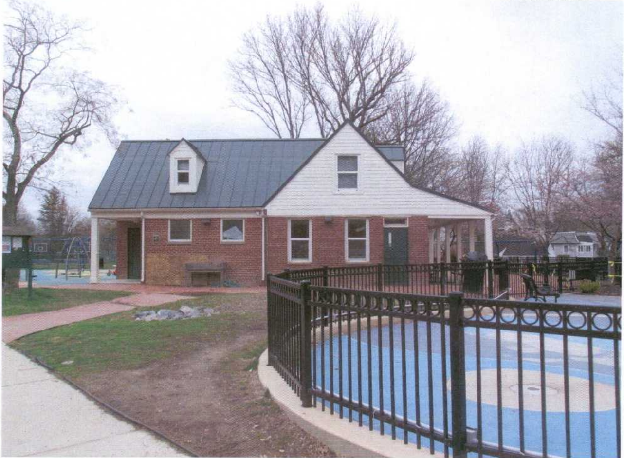
Chevy Chase Playground and Field House Washington, DC March 20, 2016 Kent Boese Chevy Chase Field House, Southwest Elevation 9/15
