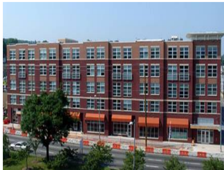
The Grays on Pennsylvania Avenue, SE
