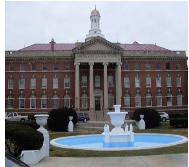
Walter Reed Old Hospital - Building #1
