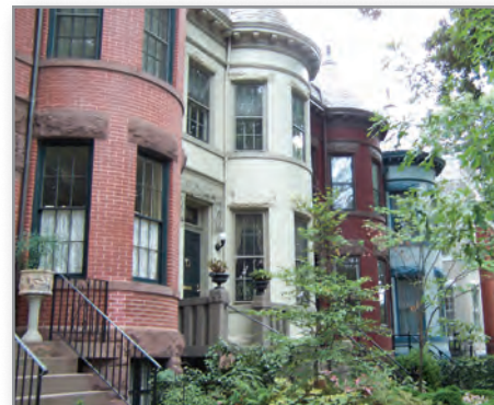
Approximately 54 percent of the housing units in the Capitol Hill Planning Area are row houses.
