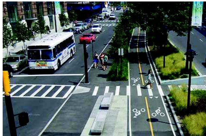
Protected Bicycle Track
