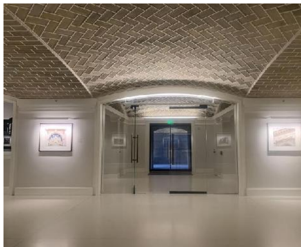
Figure 18: Guastavino tile ceiling, basement gallery, looking south. EHT Traceries, 2019.
